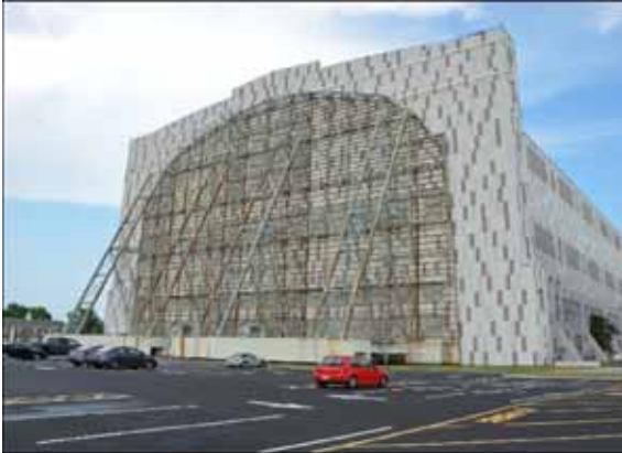
Fig. No. 8: Hangar No. 1, Lakehurst. 16
