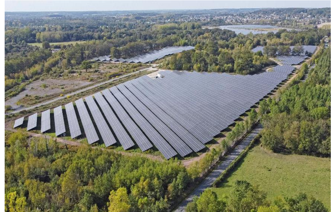
LoirecoPark – 39 MWp – France
