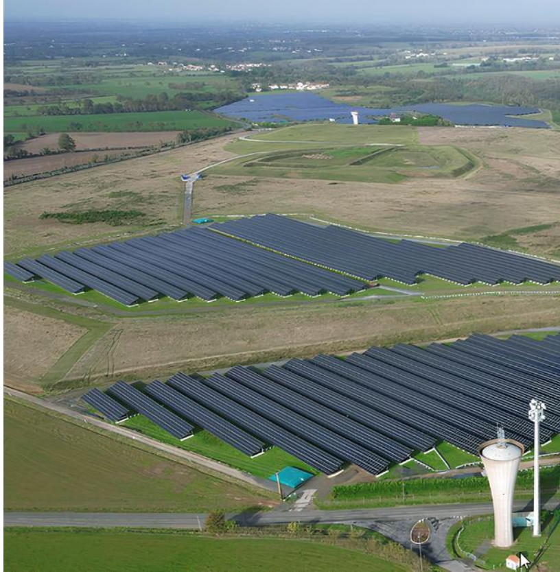
Ecarpière – 15 MWp – France
