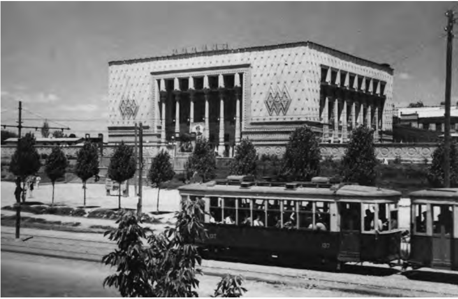
The newly constructed Vatan/Rodina theater, 1930s. Courtesy Russian State Archive of Film and Photodocuments, Krasnogorsk, Russia
