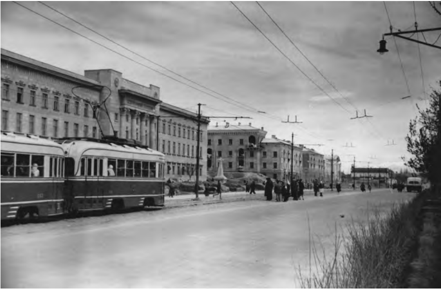
Construction site in Tashkent's New City area. Courtesy Russian State Archive of Film and Photodocuments, Krasnogorsk, Russia
