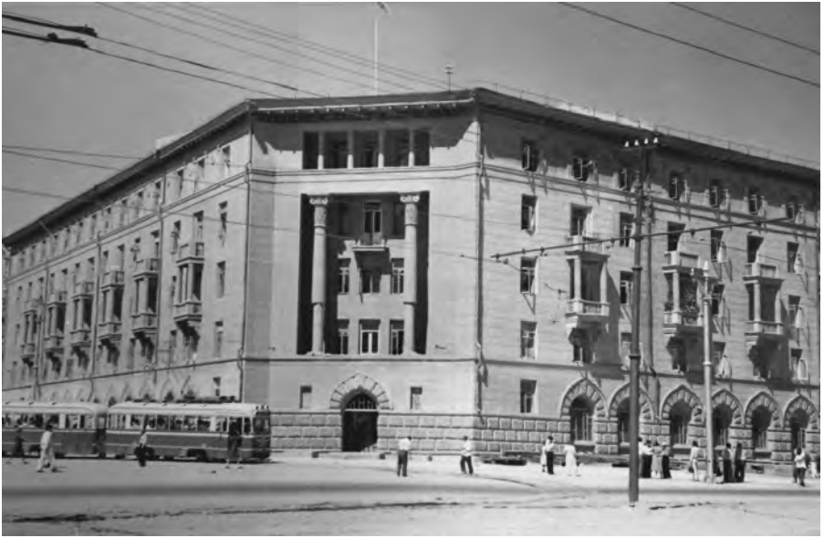
Navoi Street intersection where Uzbek-Soviet architecture can be seen. Courtesy Russian State Archive of Film and Photodocuments, Krasnogorsk, Russia
