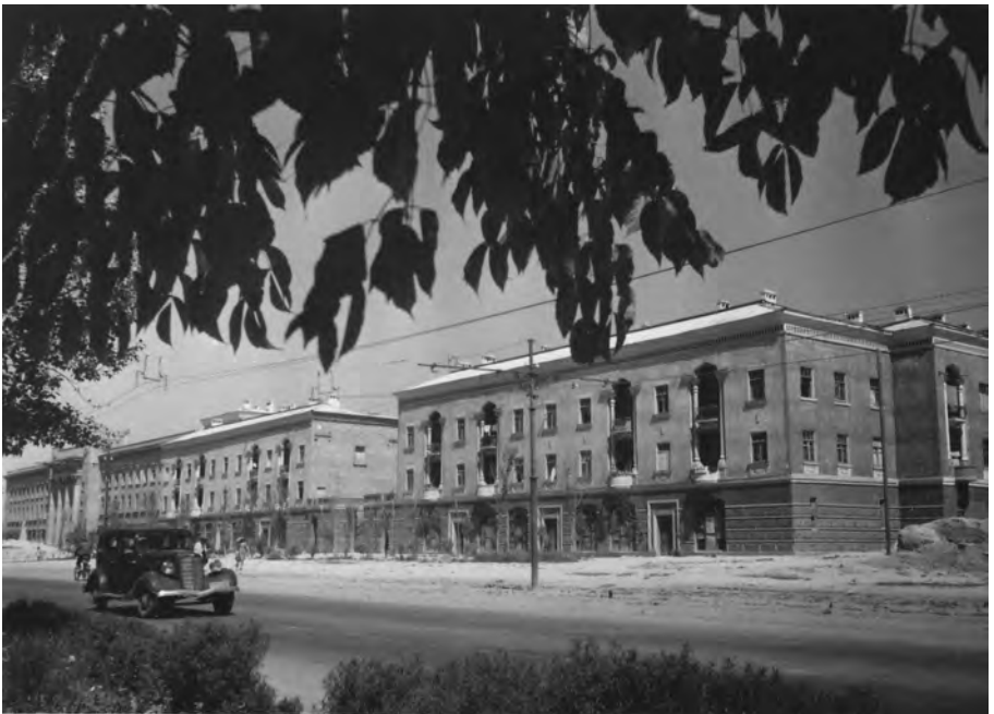
Navoi Street housing and retail construction with newly strung electric lines, mid-twentieth century. Courtesy Russian State Archive of Film and Photodocuments, Krasnogorsk, Russia
