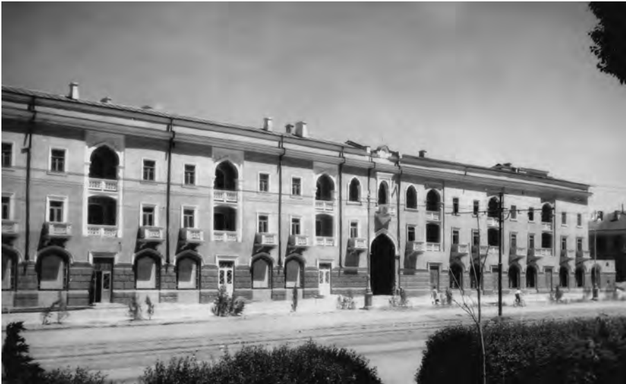
Uzbek-Soviet architecture in central Tashkent, featuring lancet arches as well as light-colored stucco to deflect sunlight. Courtesy Russian State Archive of Film and Photodocuments, Krasnogorsk, Russia
