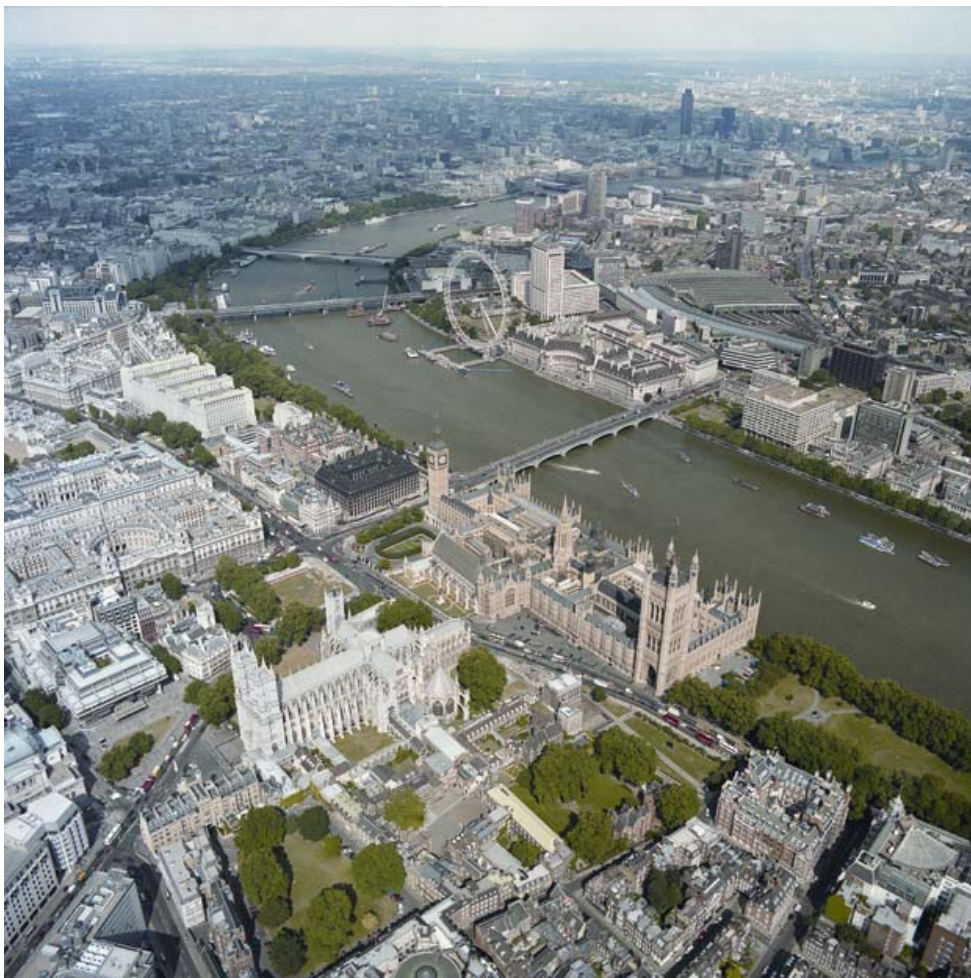
Aerial view of Westminster, with the L-shaped Jewel Tower sitting behind 7 Palace Yard in between Westminster Abbey and the Houses of the Parliament
