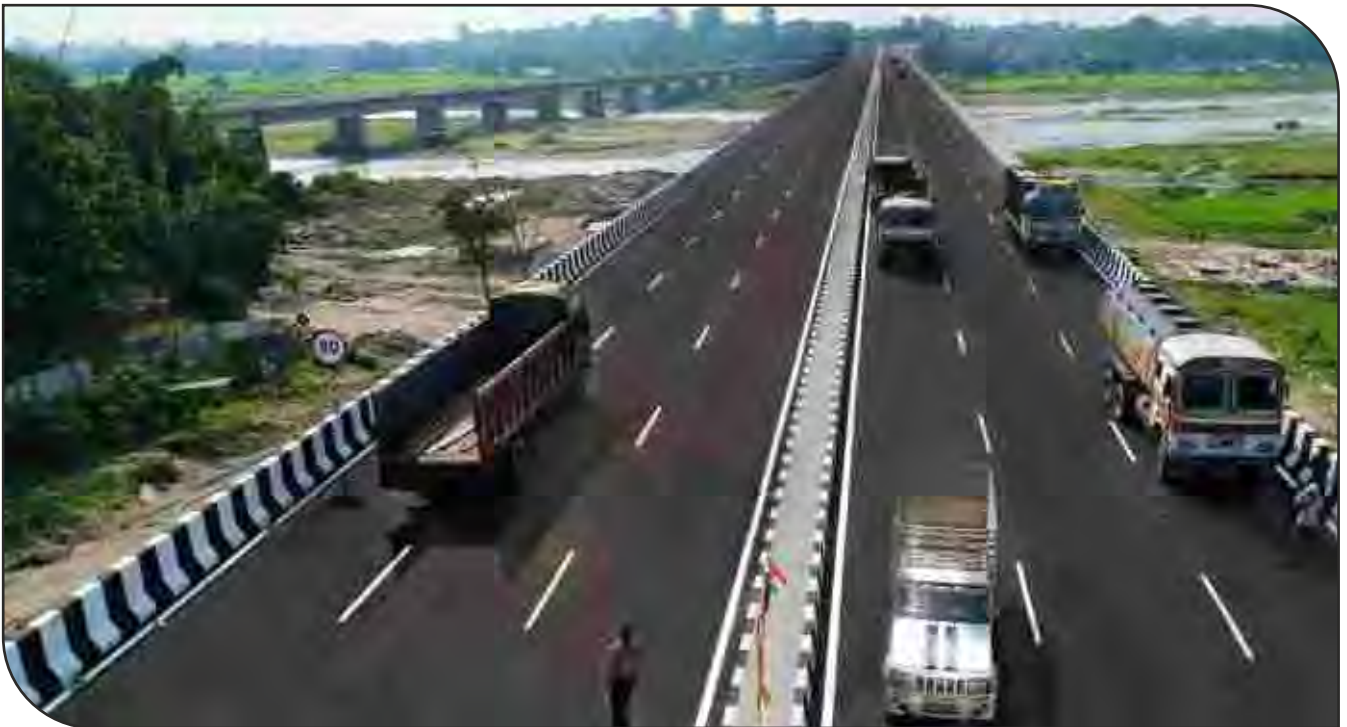
Mechi River Bridge
