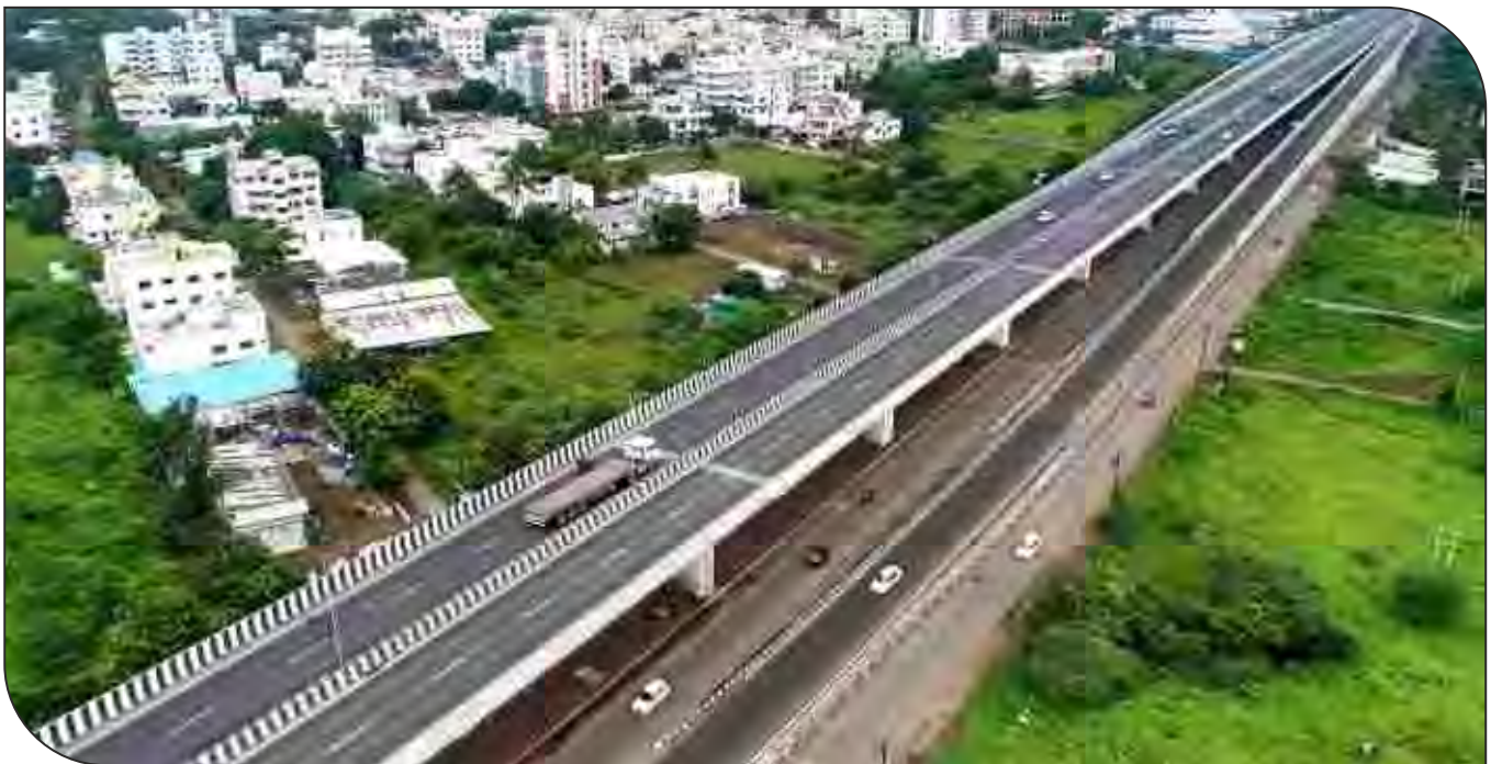
New elevated corridor in Nashik city on NH-60
