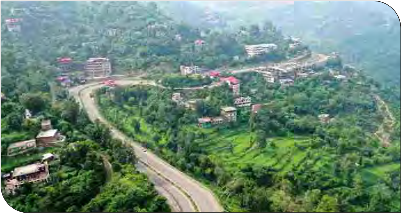
Parwanoo-Solan section of Nh5
