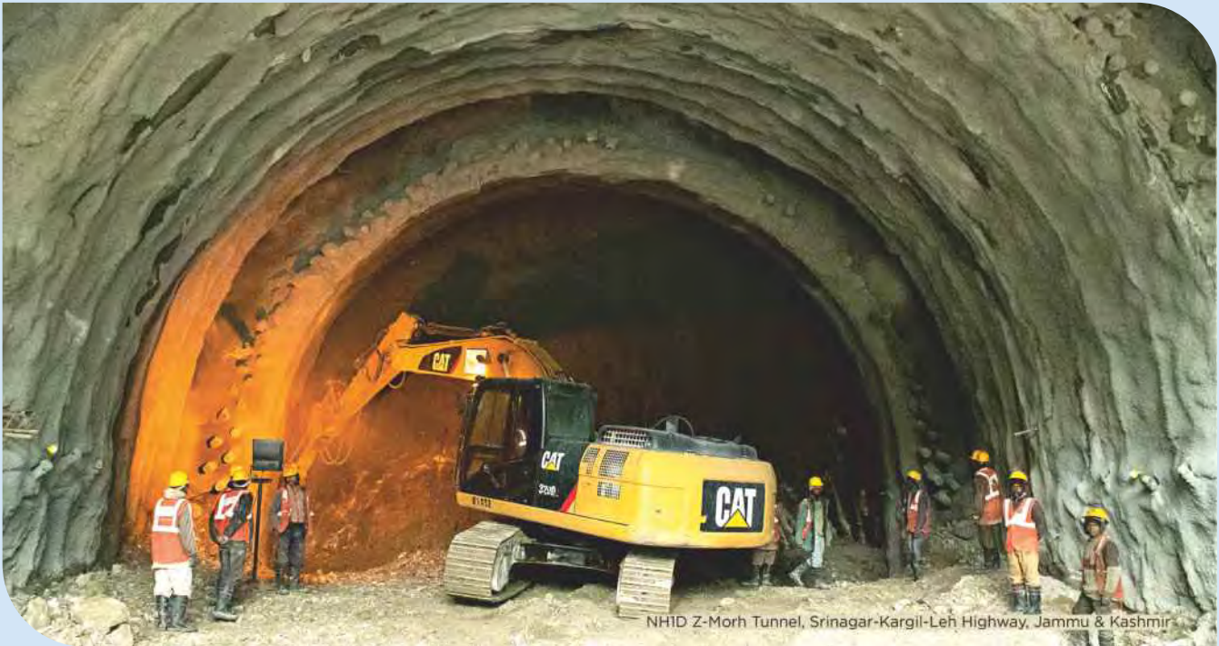
NH1D Z-Morh Tunnel, Srinagar-Kargil-Leh Highway
