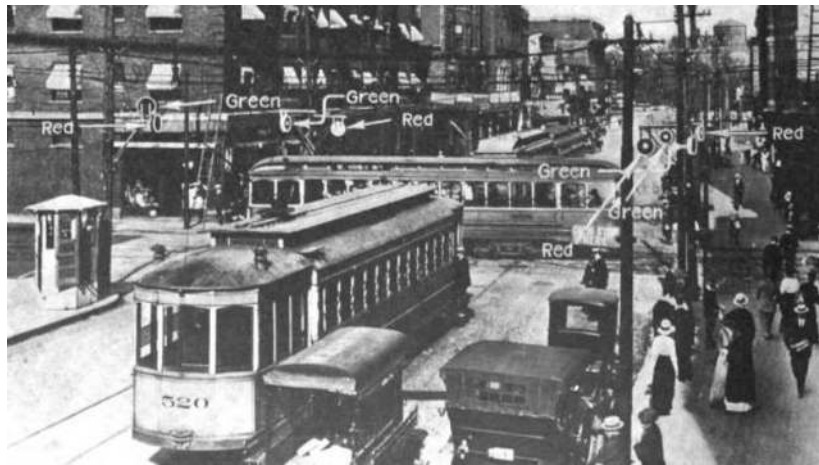
Figure 5.5.: A picture of old traffic lights (1914). Source: Vox.
