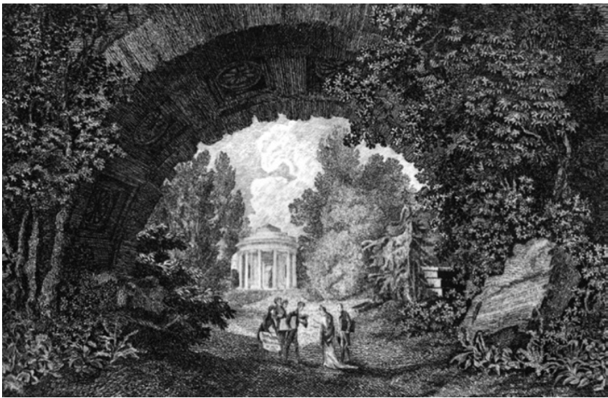
PLATE 30.13 Temple of Diana framed by the 'ruined' 'Greek' Arch at Arkadia (Collection James Stevens Curl).
