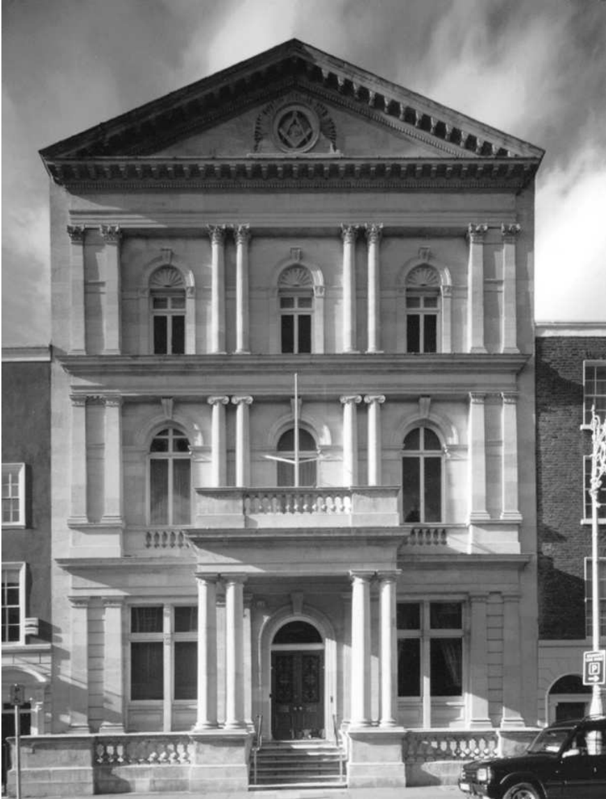
PLATE 30.27 Exterior of Freemasons' Hall, Molesworth Street, Dublin, showing the superimposed Orders (Image reproduced by permission of The Grand Lodge of Freemasons of Ireland).
