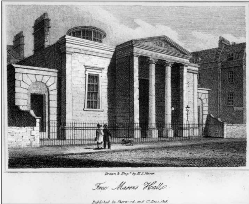
PLATE 30.23 Freemasons' Hall, Bath, Somerset, by William Wilkins, again showing the in antis arrangement of columns in a Greek Revival building (United Grand Lodge of England).
