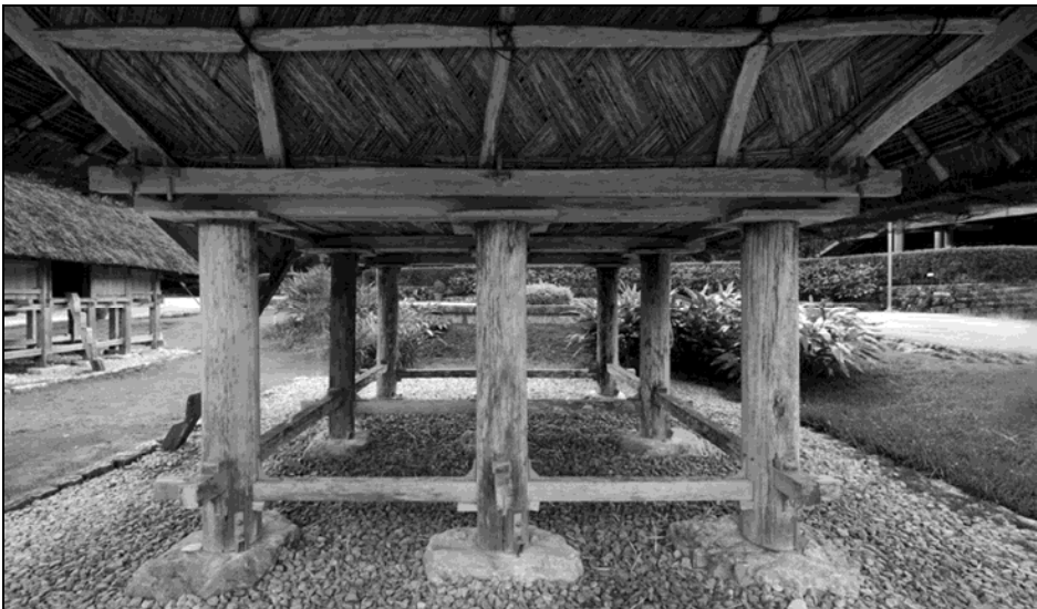
Figure 8. Nine-pillar Okinawan Granary (photographed by Hiro Kurashina). Square wooden plates atop the wooden pillars serve as rat-guards.
