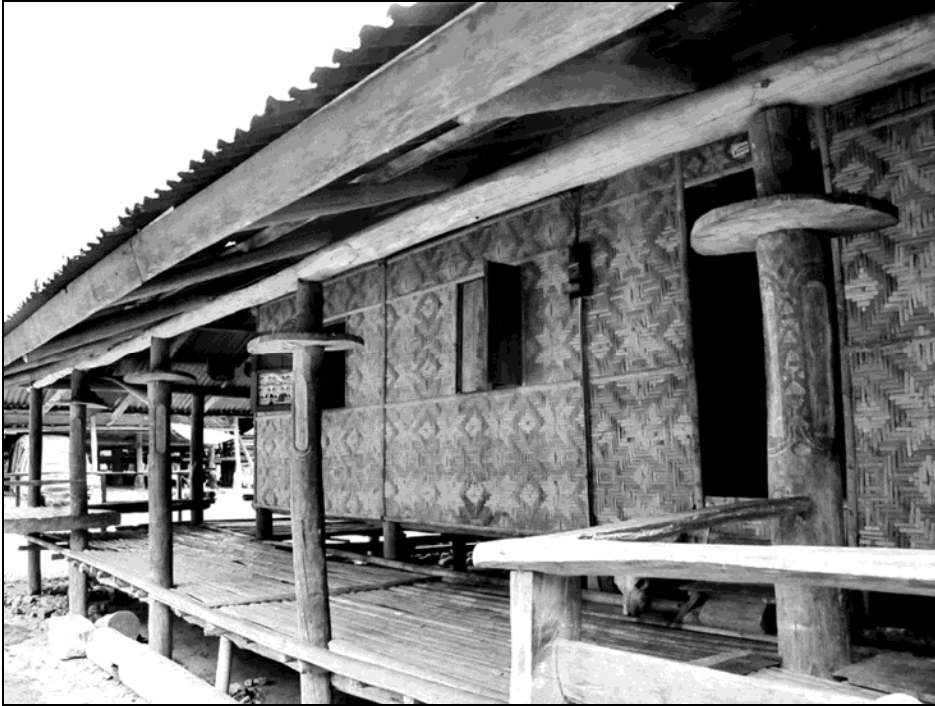
Figure 10. Rat-guards in the form of thin circular wooden discs near the top of carved wooden posts that support the horizontal beam below the roof at a traditional house in Anakalang, West Sumba, Indonesia (photographed by Hiro Kurashina in May, 2010). The thatched roofs are replaced by corrugated tin roofs in some of the modern houses observed.
