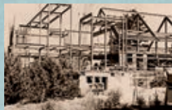
Fall 1988 Construction begins
