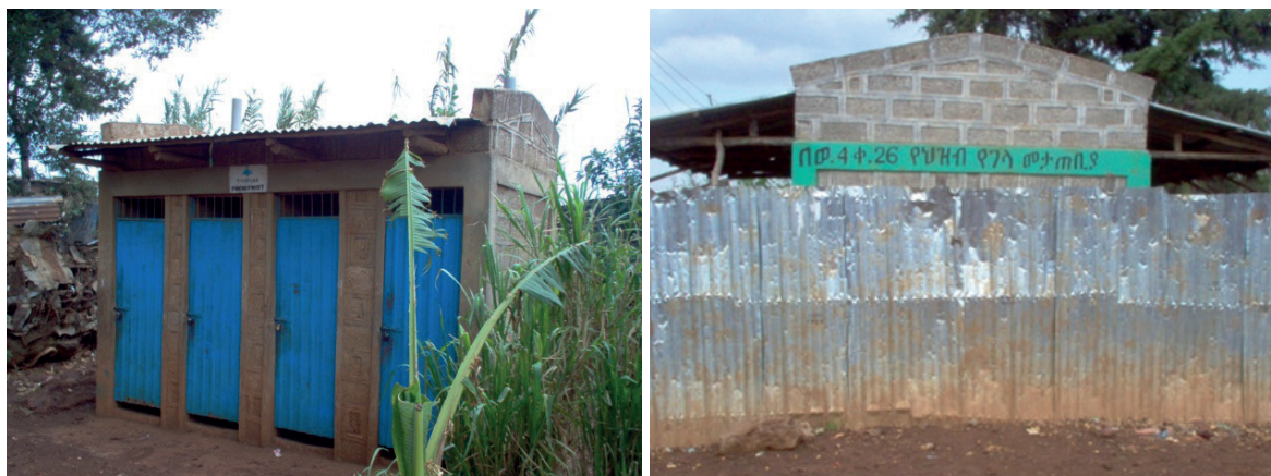
Figure 5 Upgrading of toilets and public showers
