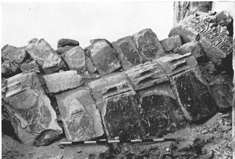
A: Fallen pier from south-west corner of inner wall.
