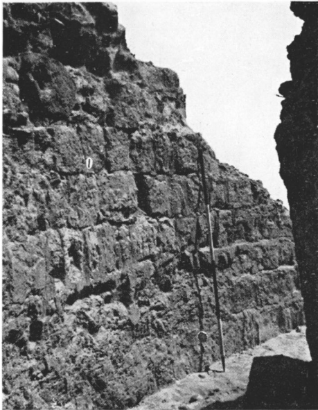
A: The space between the circular walls on the middle terrace.
