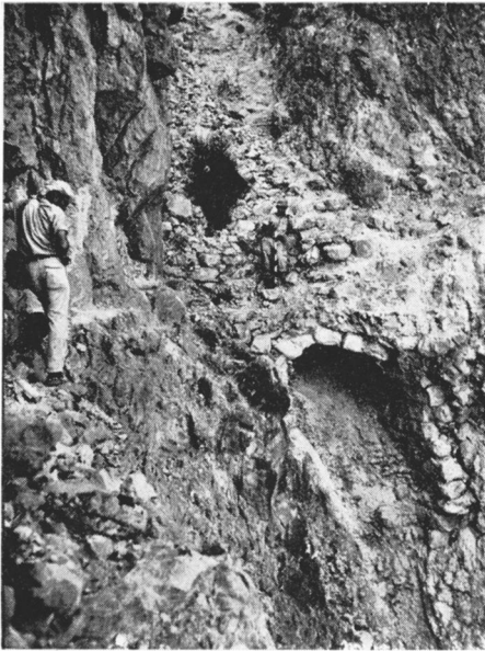
A: Vaulted arch of aqueduct.
