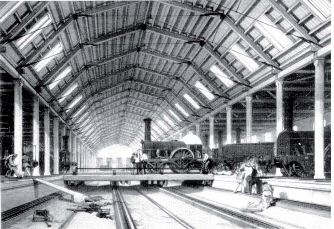
Great Western Railway Company, veturhalli, Swindon 1830.
