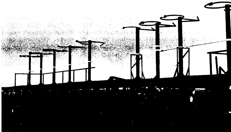
Figure 3.-Runway 35L ILS localizer antenna.
