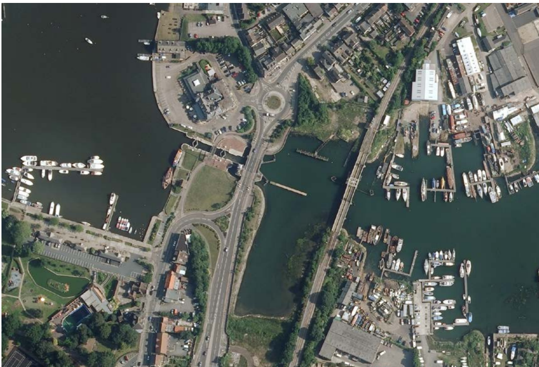
Figure 2-14: Lifting bridge and railway swing bridge at Mutford Lock, at the western end of Lake Lothing
