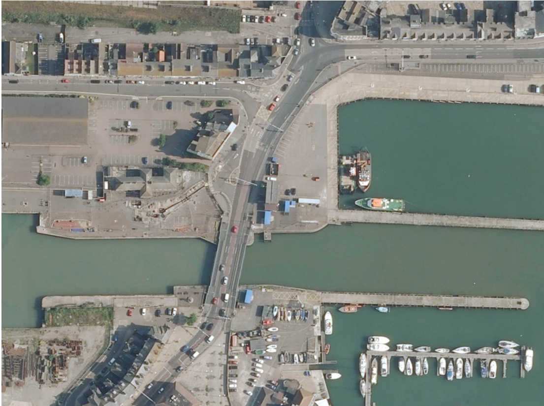
Figure 2-13: Bascule Bridge at the eastern end of Lake Lothing
