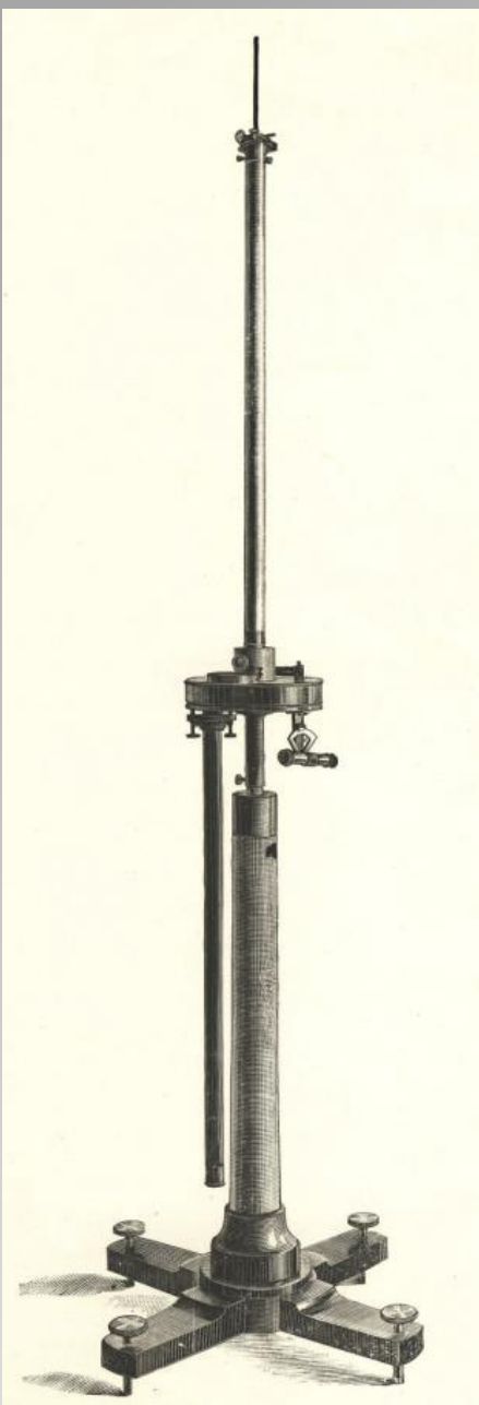
First Eötvös torsion balance: Horizontal variometer , 1890
