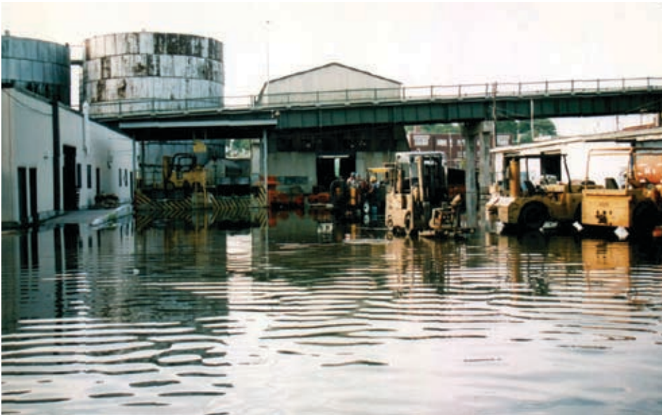
If a declaration is made by a floodplain administrator that a facility is substantially damaged, a determination must be made quickly regarding actions that will need to be taken to make repairs, or whether the facility must be replaced.
