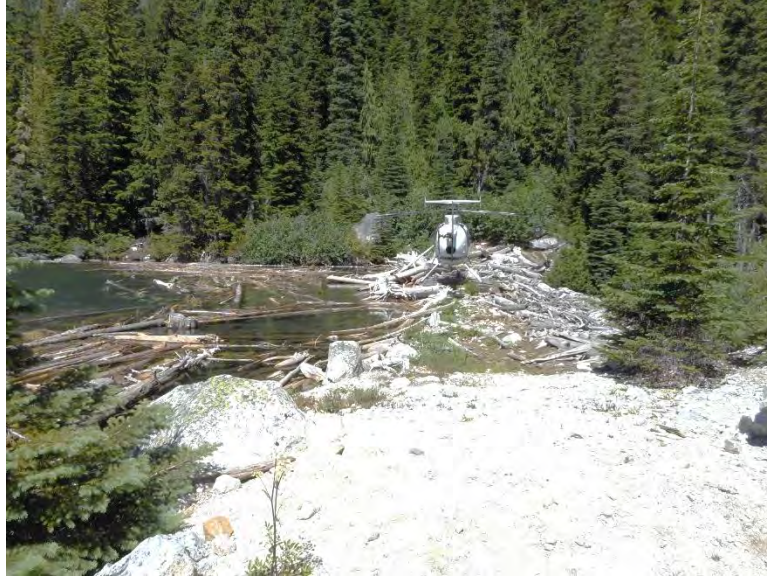
Photo 12 – Lower Klon aqua Dam Embankment, View along Crest from South
