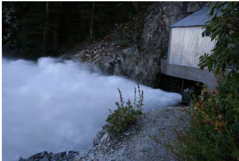
Photo 36 - Upper Snow Lake Outlet Works – Discharging to Nada Lake
