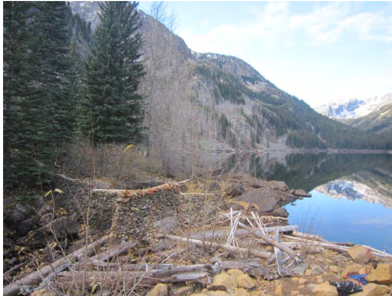
Photo 14 - Eightmile Lake Dam (Submerged Gate Not Visible)
