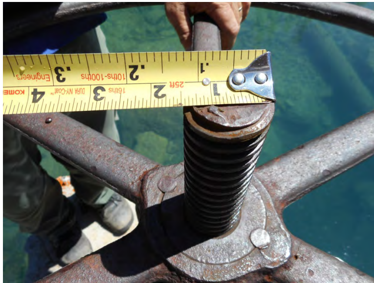
Photo 20 - Colchuck Lake Gate Actuator Stem (After Operation)
