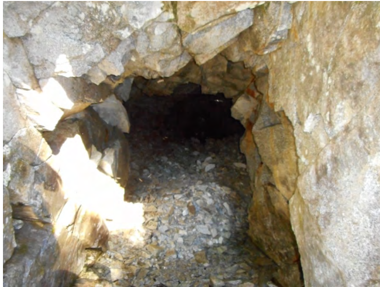
Photo 3 - Square Lake Entrance to Outlet Works Tunnel
