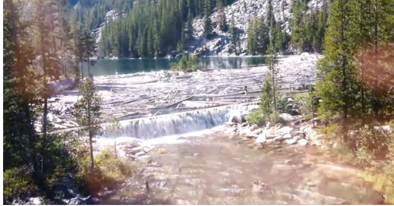
Photo 25 - Upper Snow Lake Dam and Spillway during Spill, Aerial View
