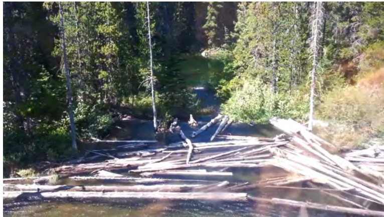
Photo 27 - Lower Snow Lake Dam, View from Lower Snow Lake Side
