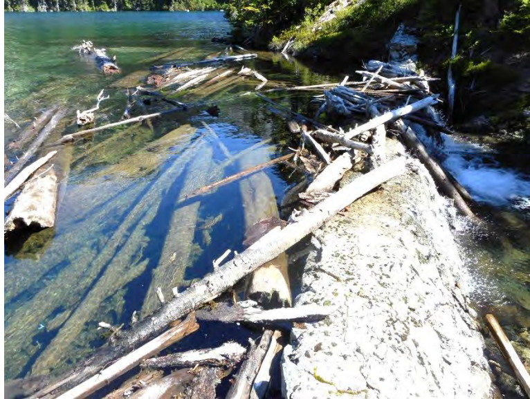
Photo 7 - Square Lake Dam along Crest
