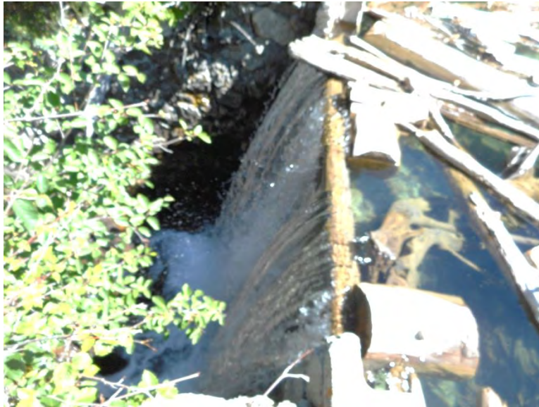
Photo 23 - Colchuck Lake Dam Spillway with Stop-Logs in Place
