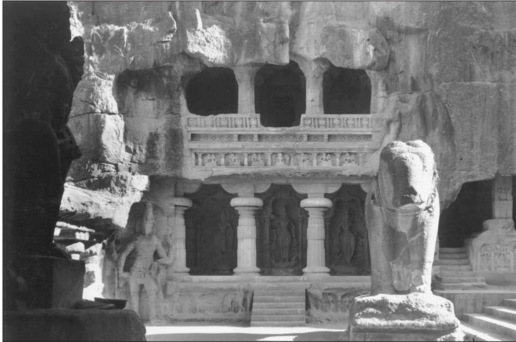
The Kailasanatha Temple in the state of Maharashtra is surrounded by artificial caves sculpted into solid rock.
