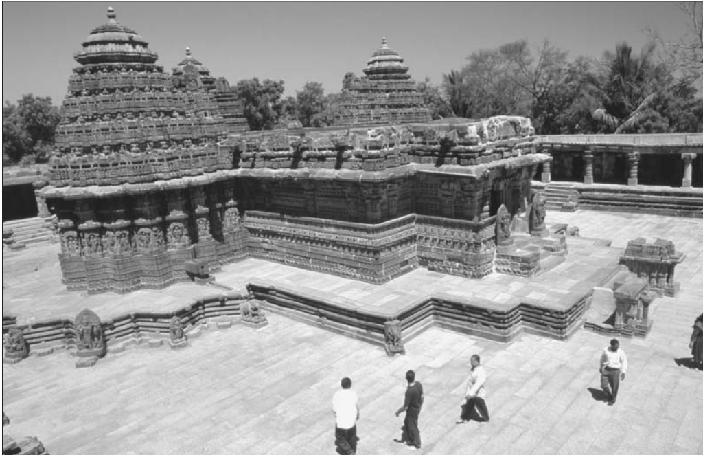
The Shri Channakeshara temple in Somnathpur, India. A traditional feature of Hindu temple architecture is the adhishtana, a raised base upon which the temple is built.
