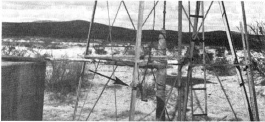
Windmill. Note windlass (arrow).
