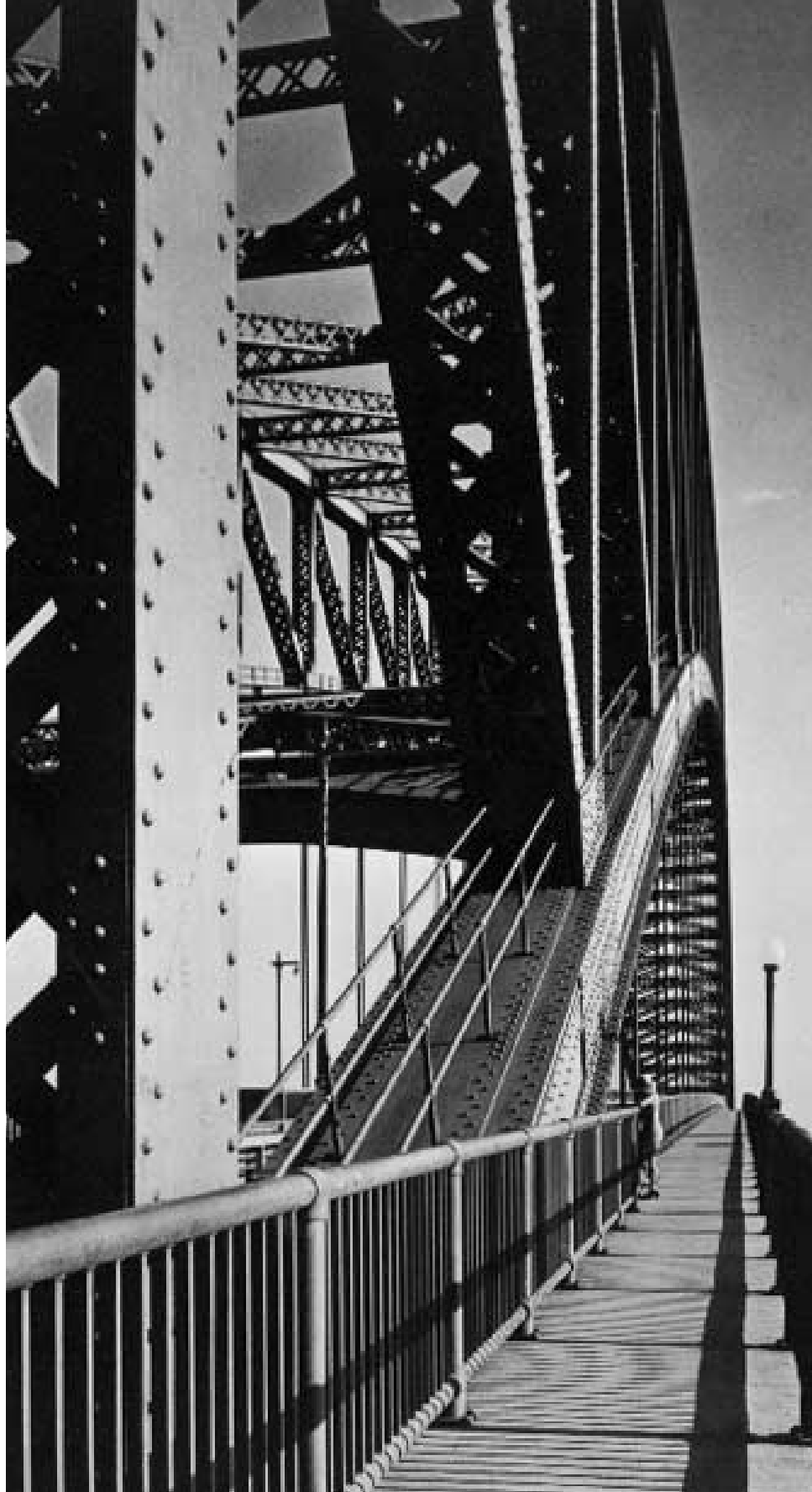
A pedestrian on the walkway in the 1930s looks toward the bridge's roadway.
