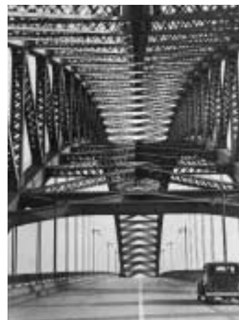
Crossing under the arch from a motorist's perspective.
