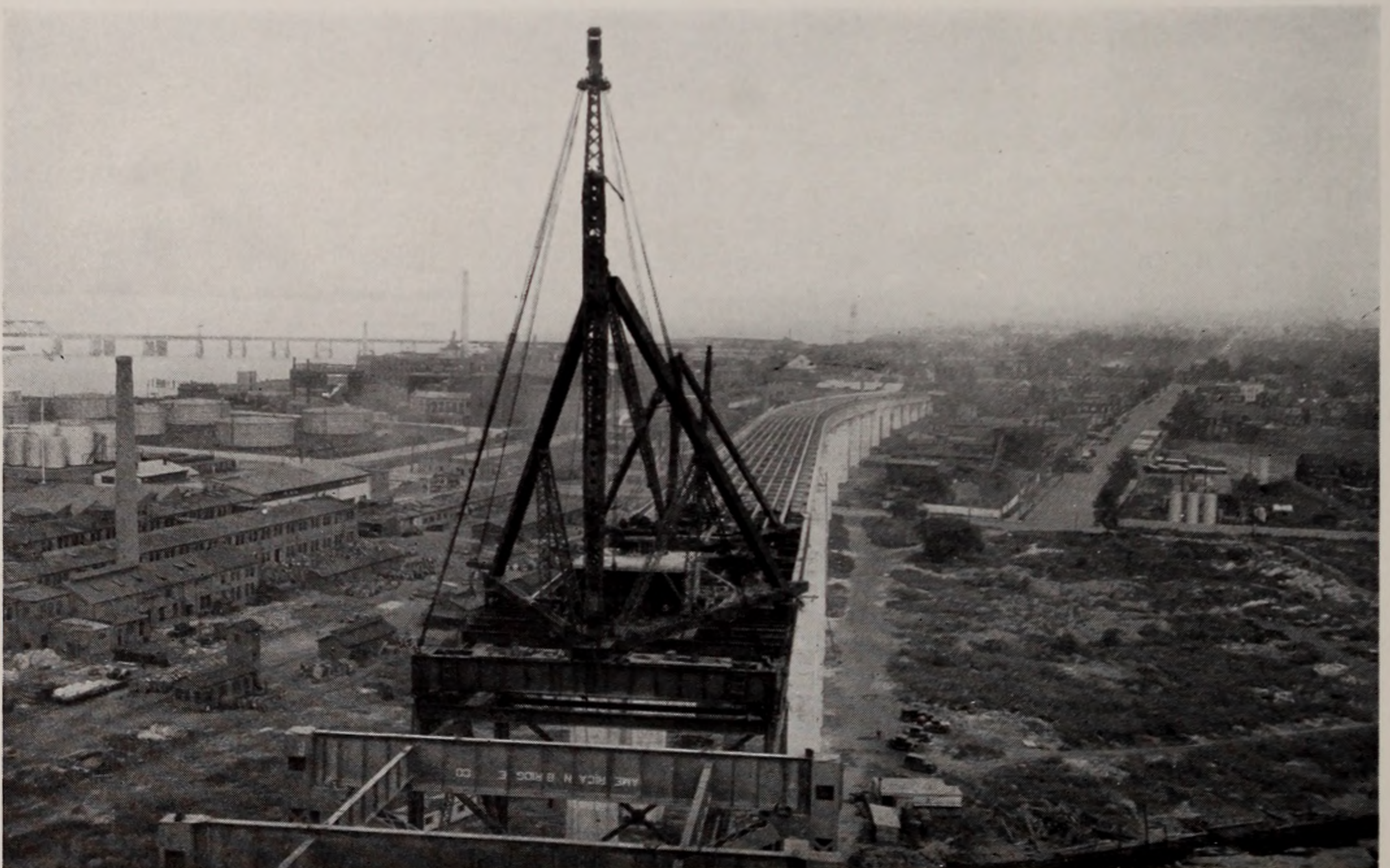
PORT RICHMOND APPROACH STEEL ERECTION. NOVEMBER 26, 1930
