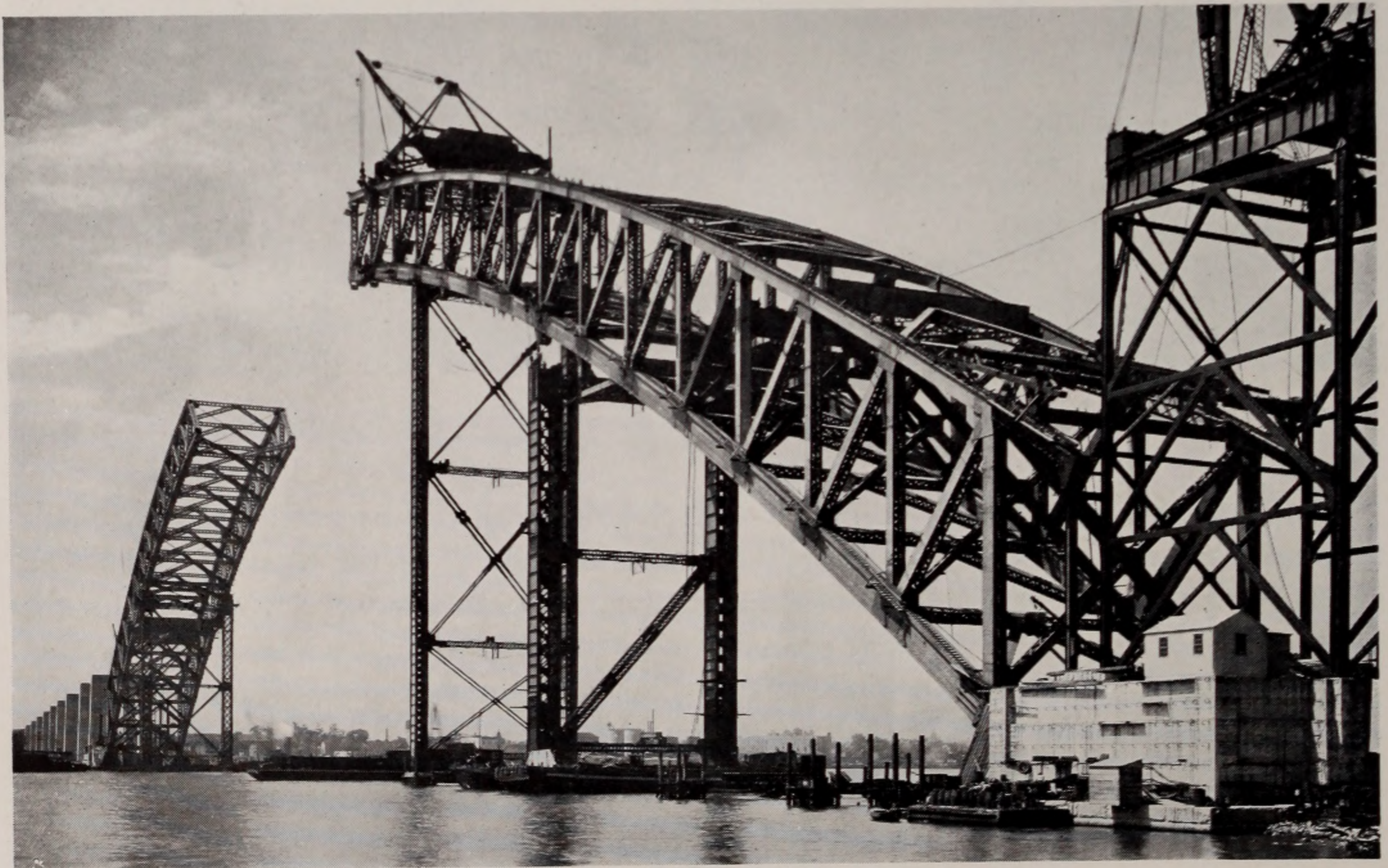
ERECTING NORTH SECTION OF ARCH, BAYONNE ABUTMENT IN FOREGROUND. JULY 15, 1930
