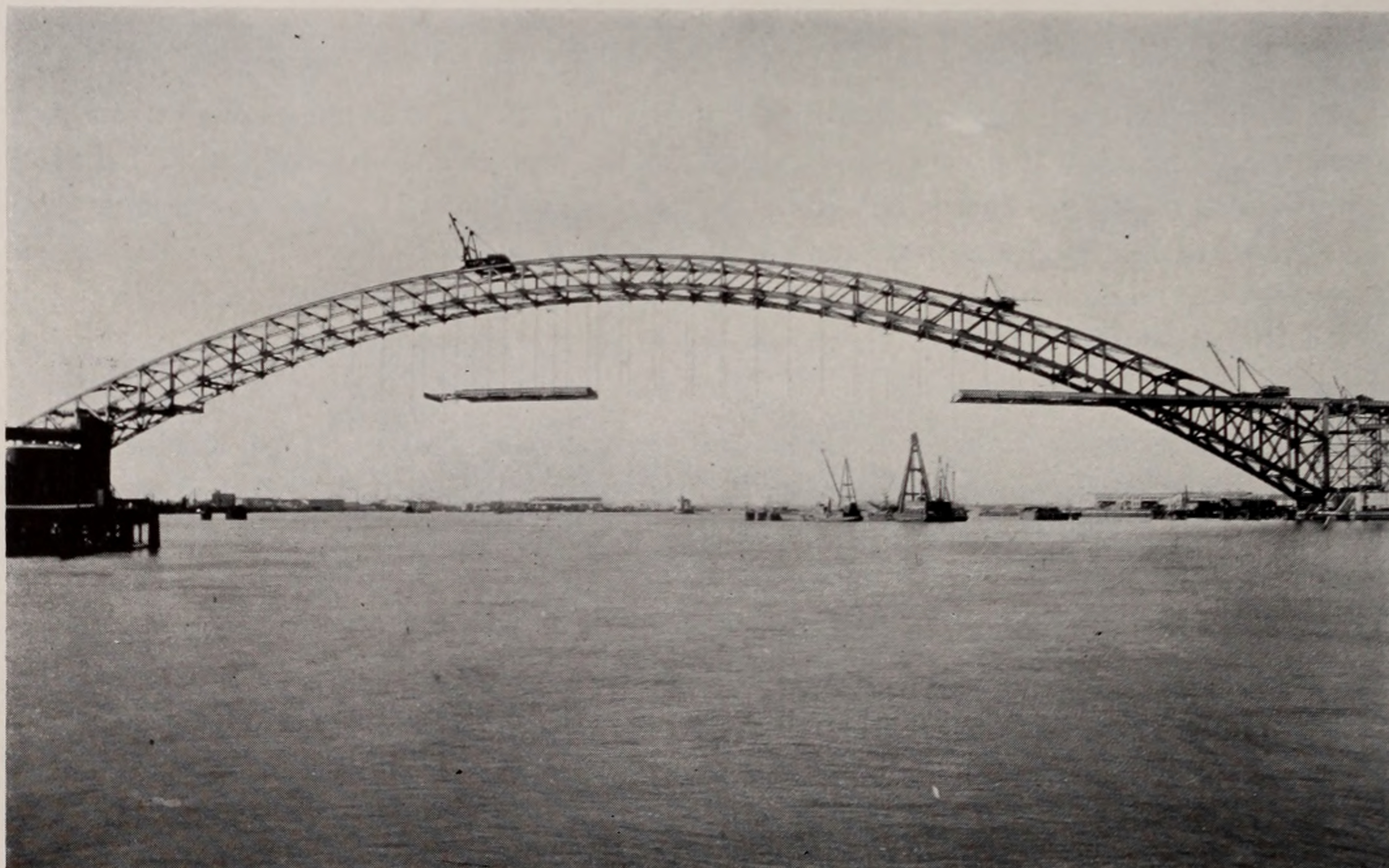
ERECTING FLOOR STEEL IN TWO SECTIONS. DECEMBER 17, 1930
