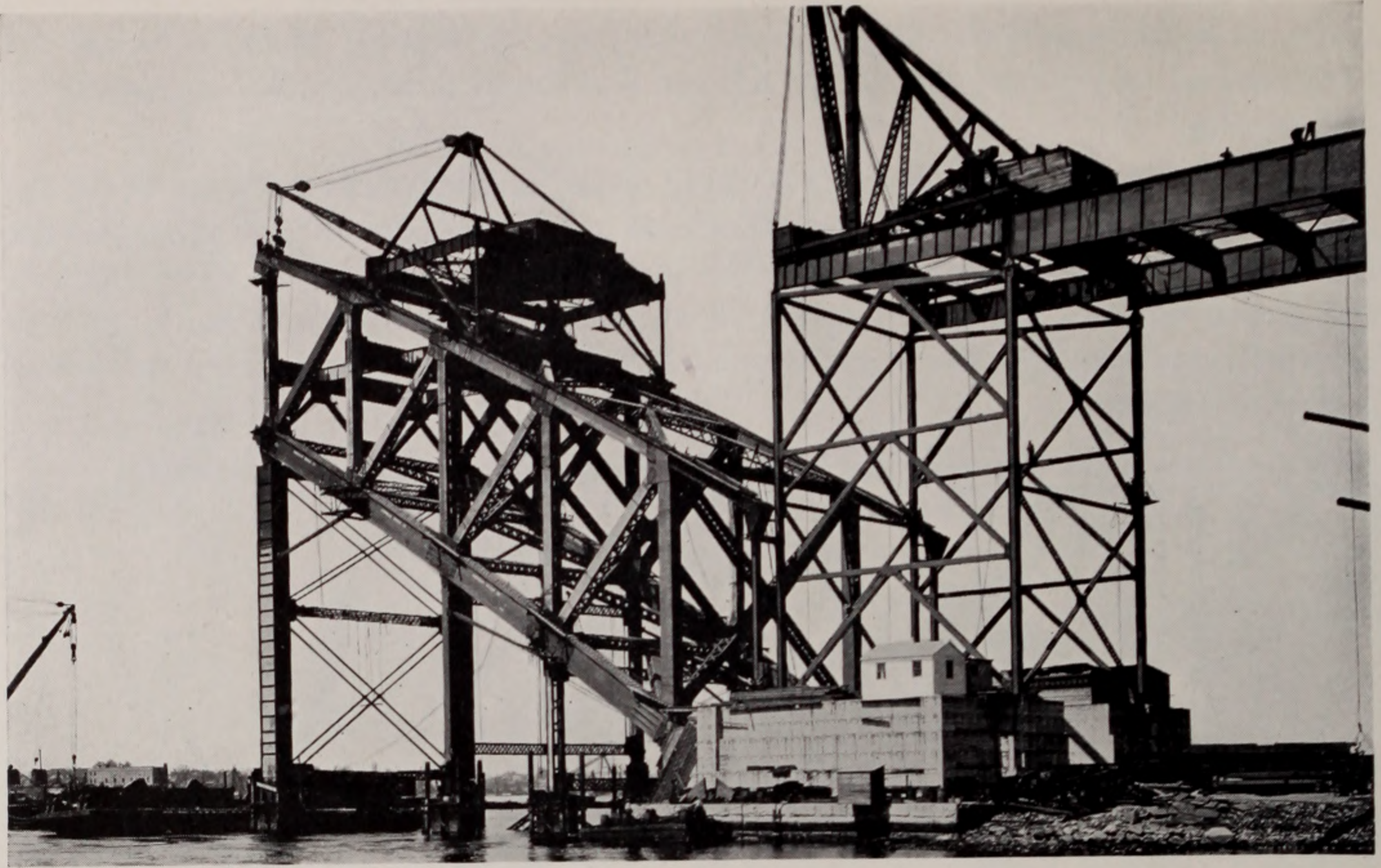
ERECTING NORTH SECTION OF THE ARCH. MAY 9, 1930
