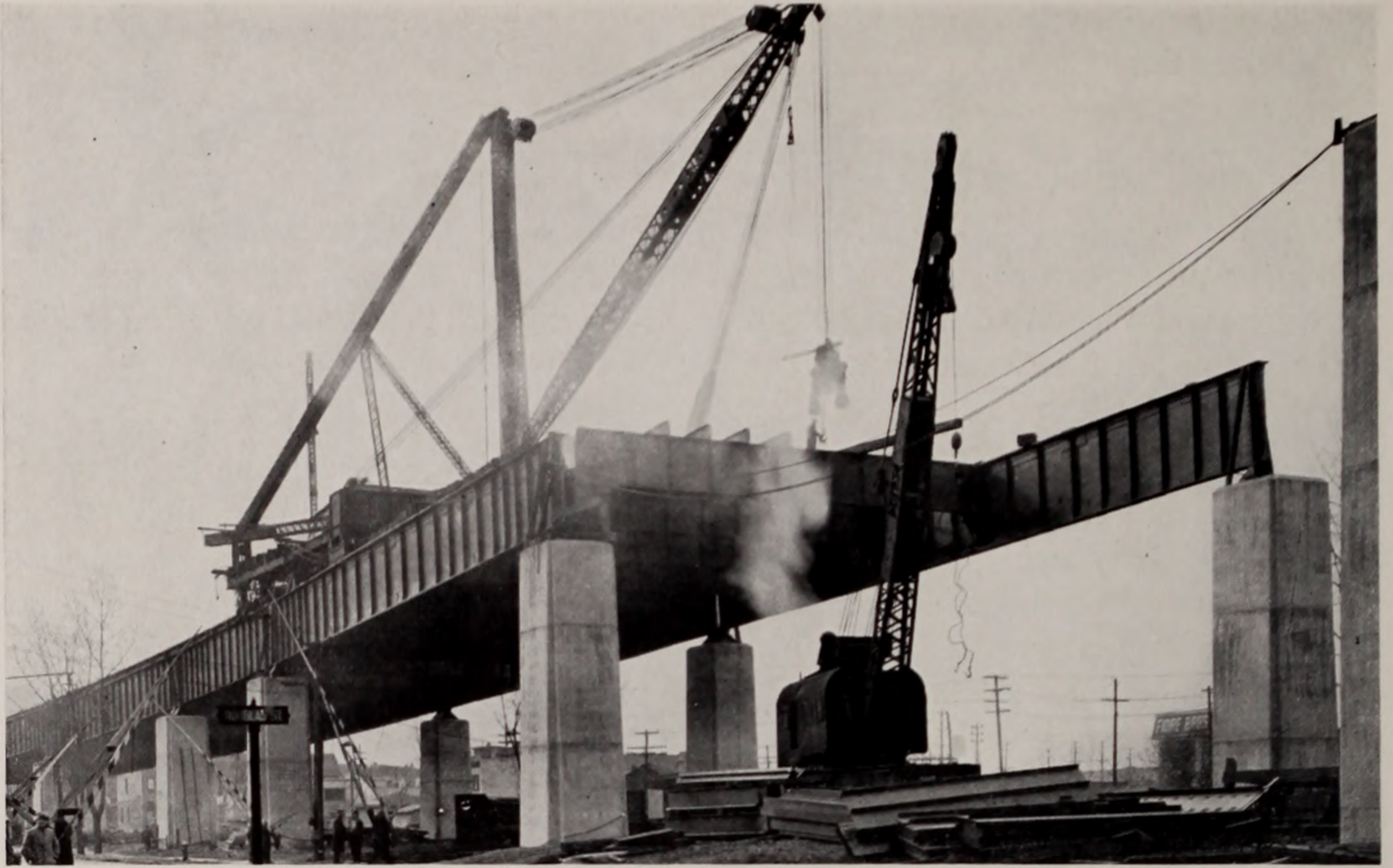
BAYONNE APPROACH FROM ABUTMENT. SEPTEMBER 18, 1930
