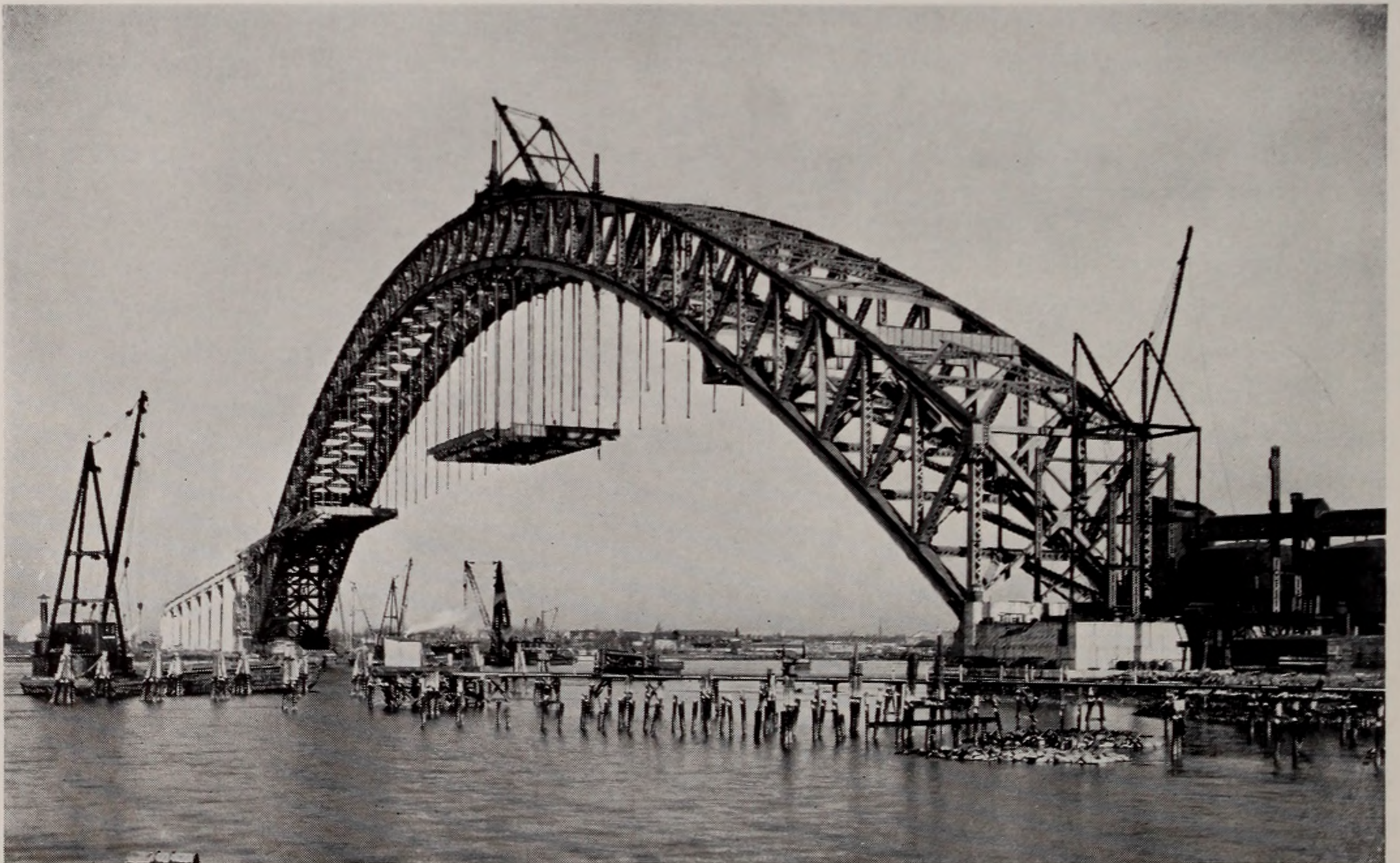
FLOOR STEEL ERECTION. PORT RICHMOND ABUTMENT IN FOREGROUND. DECEMBER 17, 1930
