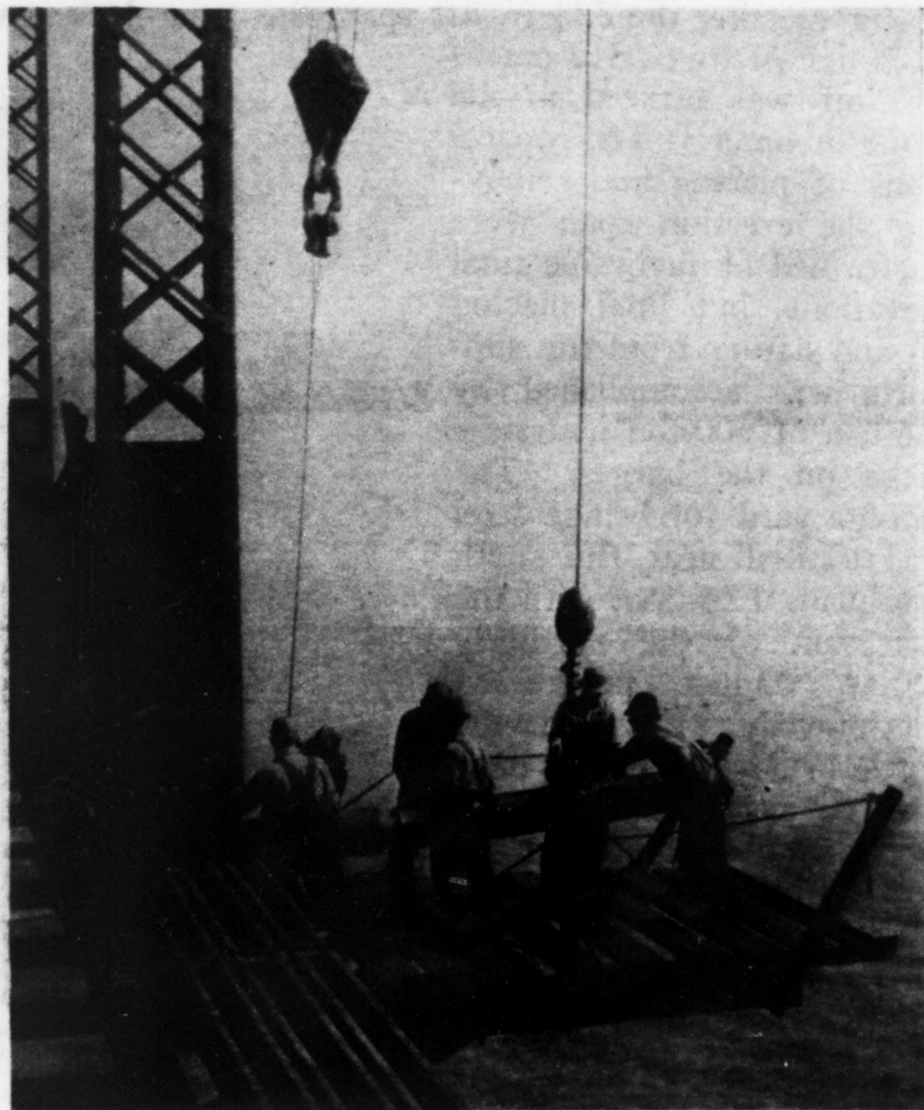
Driving pins in bottom chord
