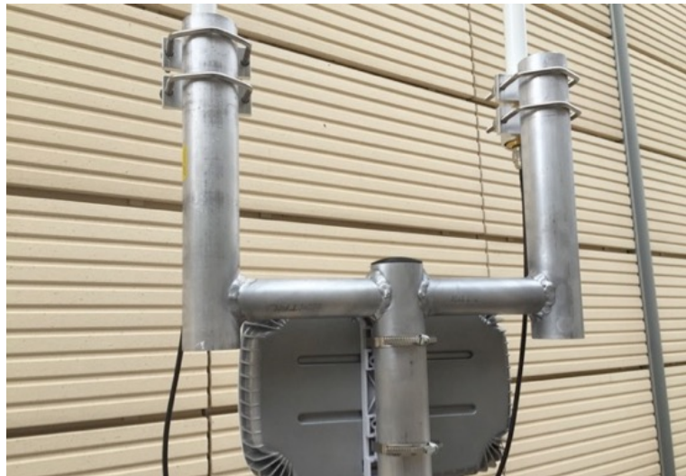
1- \lambda separated 5.5dBi 902MHz ~ 928MHz
