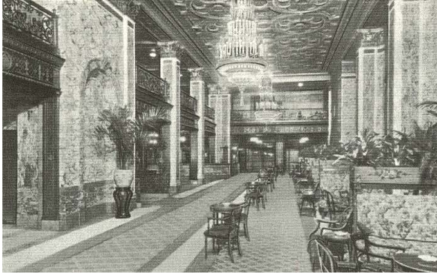
Figure 3.2: The Book-Cadillac Hotel, Detroit, circa 1930. The ostentatious ornamentation of the hotel discouraged disheveled travelers. Figure from The Motel in America , 27.
