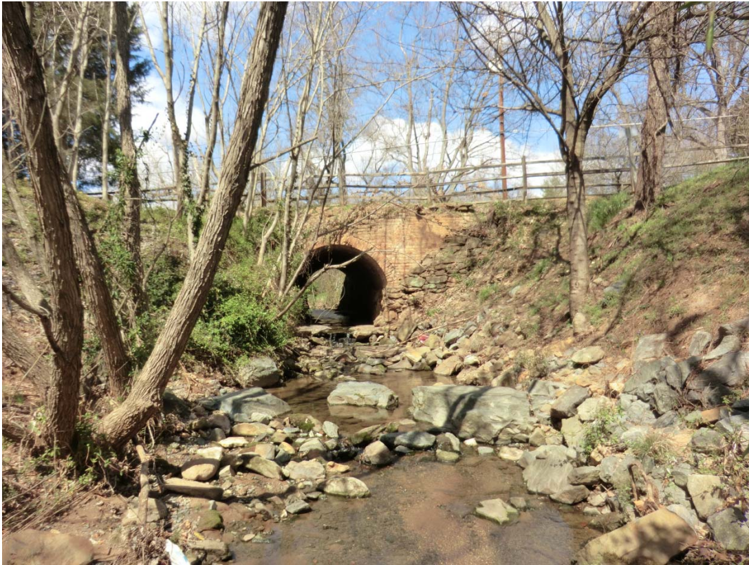
Brick barrel vault bridge over Tanners Run at Academy Street, looking north. Martha B. Hartley Photographer, April, 2013
