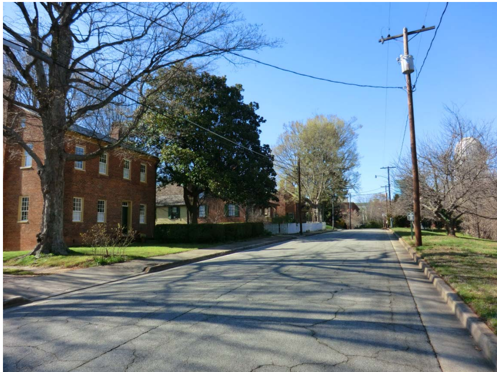
400 block of Factory Row (west side) with the Sussdorft, Ackerman and Patterson houses and Arista Mill in distance, looking north. Martha B. Hartley Photographer, April, 2013
