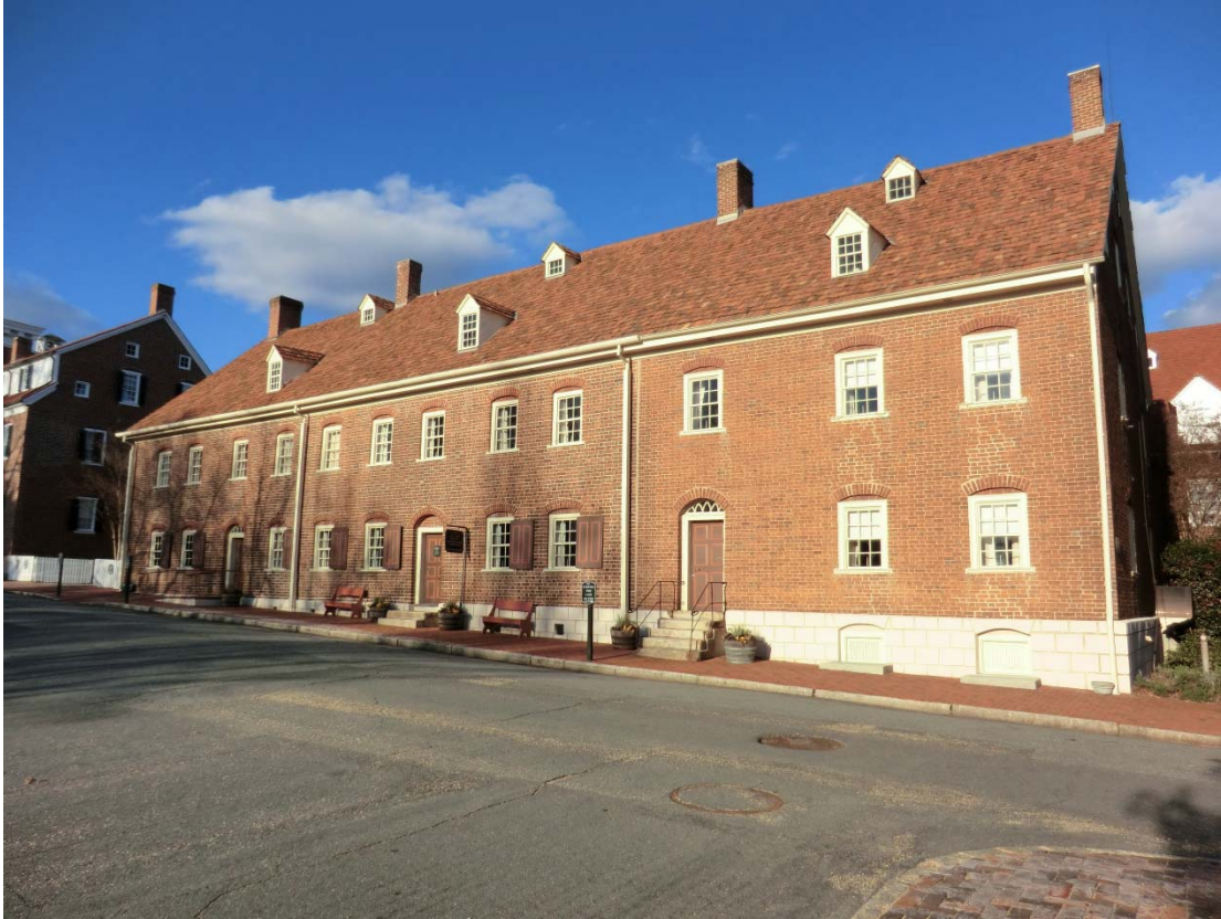
Single Sisters' House, west façade. Martha B. Hartley Photographer, April, 2013
