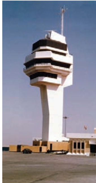
● Jebel Ali Port control tower
