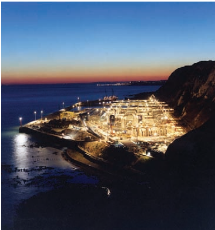
● Shakespeare Cliff Work starts on the Channel Tunnel
