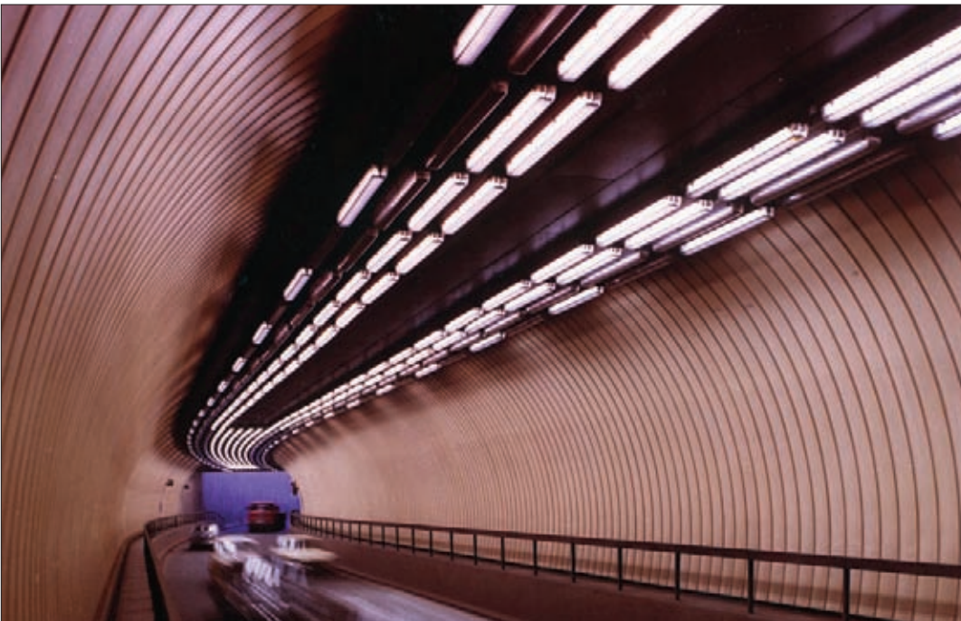
● Blackwall Tunnel Construction of the £5.3M second bore was completed in 1967
