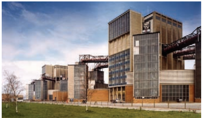
● 1957 Work starts for the new Berkeley nuclear power station
