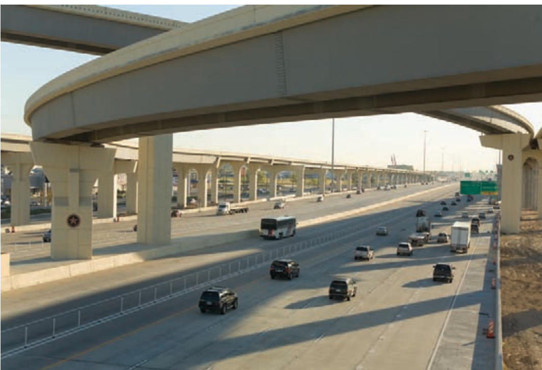
● I-10 Freeway Texas Parsons Brinckerhoff was the engineer for this £310M reconstruction project
