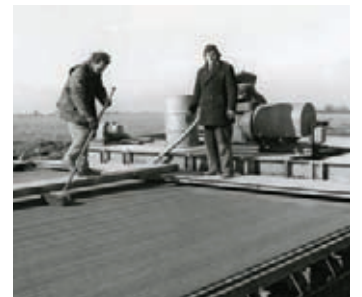
● 1979 Concreting at RAF Cottesmore
