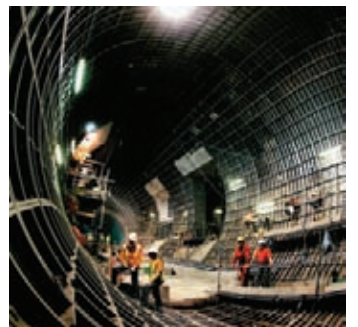
● Tunnelling Jubilee Line Extension
