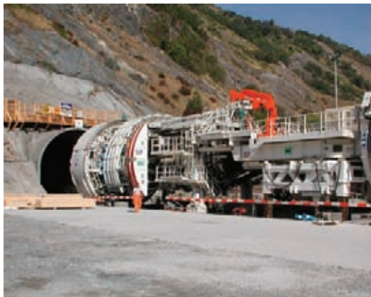
● Gotthard Base Tunnel The world's longest rail tunnel
