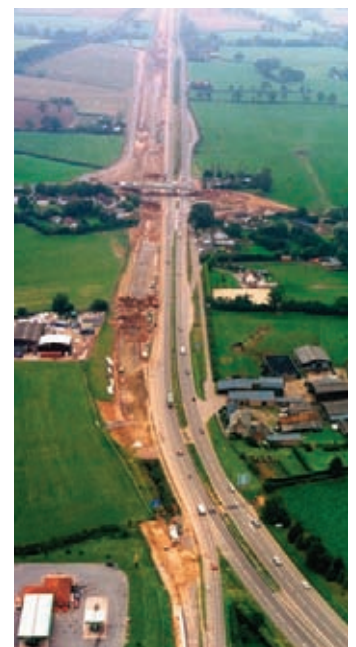
● Roads The A30/35 PFI project
