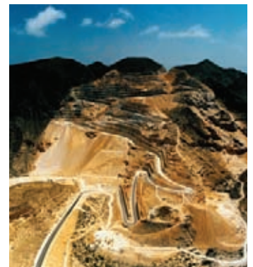
● Oman Road project at Mughsayl
