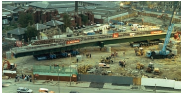
● Docklands Light Railway Bridge roll-out at Limehouse in East London
