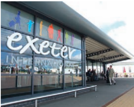
● Exeter airport A Balfour Beatty asset
