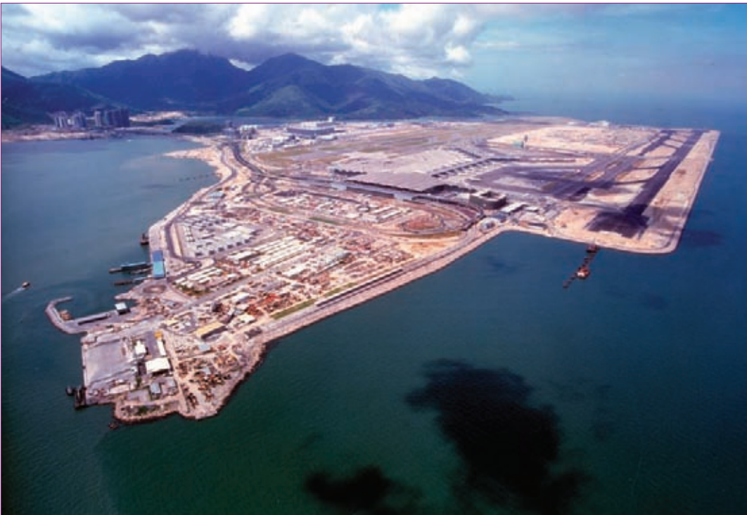
● 1998 Chek Lap Kok airport in Hong Kong opened. Balfour Beatty built the £830M terminal
