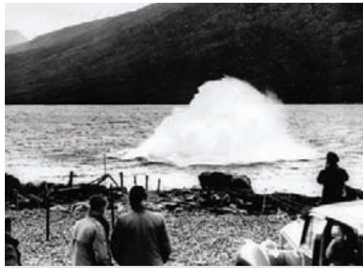
● Lochaber Underwater blast helps tunnel breakthrough
