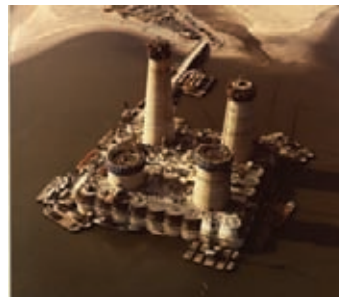
● Offshore Oil platform construction
