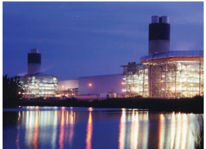
● Power Barking Power station, an early Balfour Beatty PFI scheme
