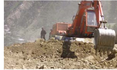
© Chaudhry Khawar Road repair, Kagan
