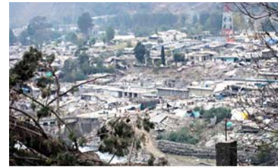
© Edge_of_Space / flickr.com Earthquake damage, Balakot
