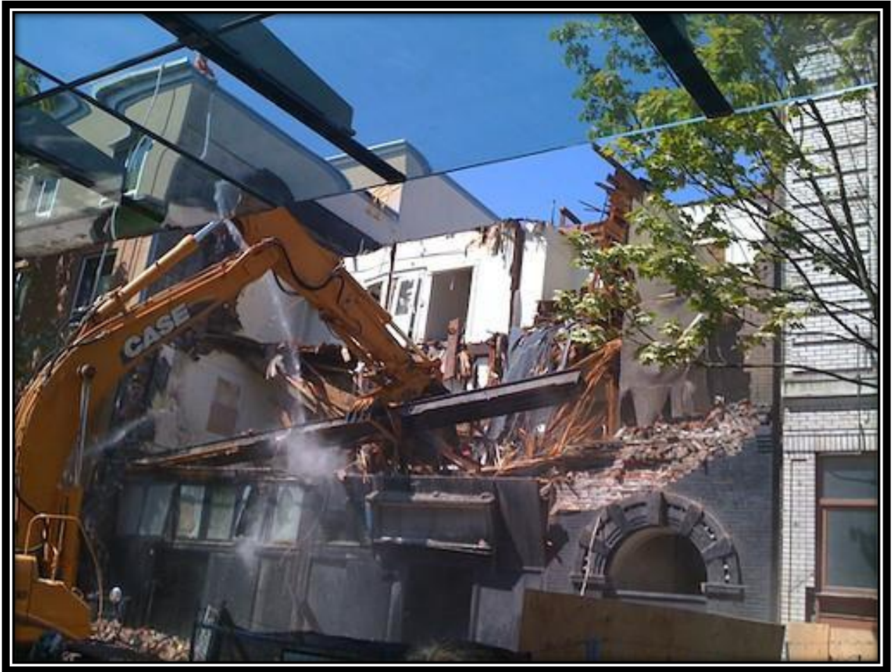
Figure 50: Demolition of the Satyricon (Oregonian Press, 2008)
