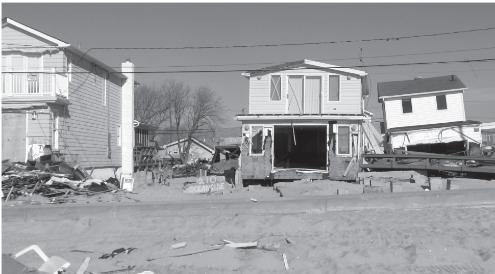
Figure 4. Flood damage caused to seafront homes in Queens, New York, by Hurricane Sandy, October 2012
