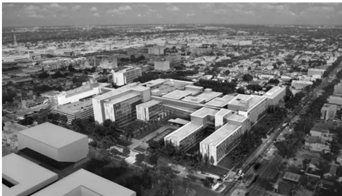
FIGURE 5.6 New Orleans Downtown Hospital Complex.
