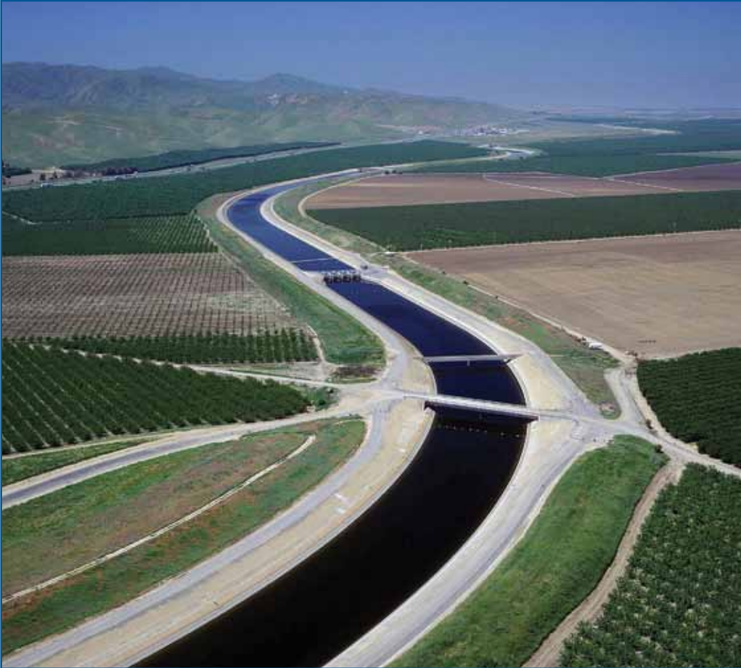
State Water Project Aqueduct, Central Valley, California
