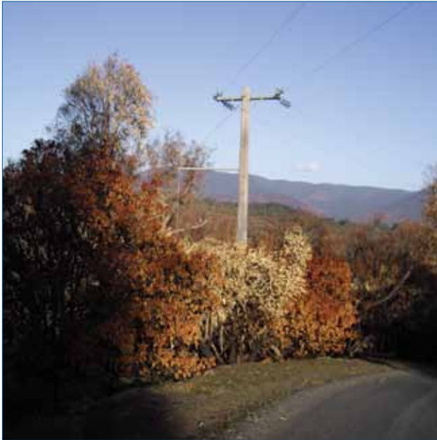
At Lake Mountain, the aftermath of the Murrindindi fire revealed pyrolyzed and gasified leaves, a result of extreme radiant heat. Photograph © Janet M. Bridgart.
