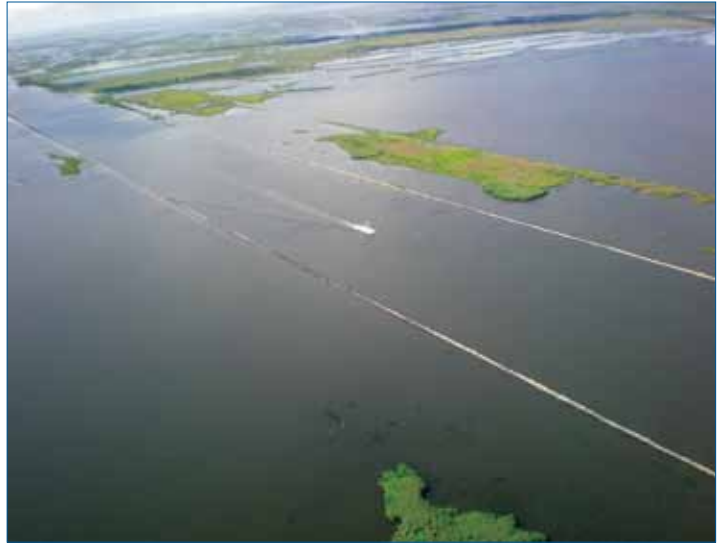
The combined effects of dredging the Mississippi River Gulf Outlet, subsequent wave energies and saltwater intrusion, and decreased freshwater and sediment supply from the Mississippi River have degraded the marsh in Breton Sound. Before its closure, protection efforts included a combination of breakwaters and shoreline rock barriers.
