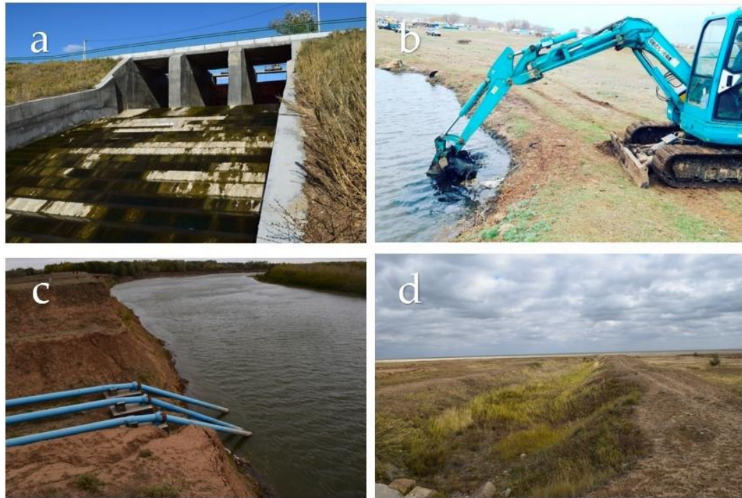
Figure 14 - Measures to restore the water content of lake Shalkar: regulated spillway from the reservoir on the river Sholak Ankaty (a); clearing of springs (b); water supply from the Ural river through the Ural-Shalkar canal, the place of water intake (c); places where the Ural-Shalkar canal flows into lake Shalkar (d)
