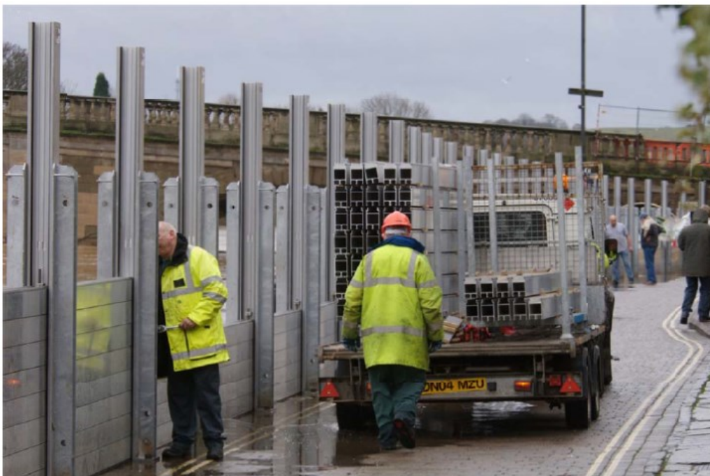
Figure 2 Demountables in action, Bewdley, Worcs, UK. Source: The Environment Agency.
