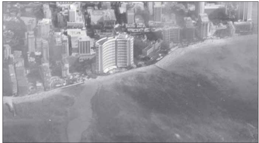
Figure 14. Halekulani, Sheraton Waikiki, Royal Hawaiian (and long curved groin), Moana Surfrider, Moana Hotels; Halekulani "sand channel" at left; aerial photo, cloudy, 30 January 1999. (By R.L. Wiegel, #9524.)
