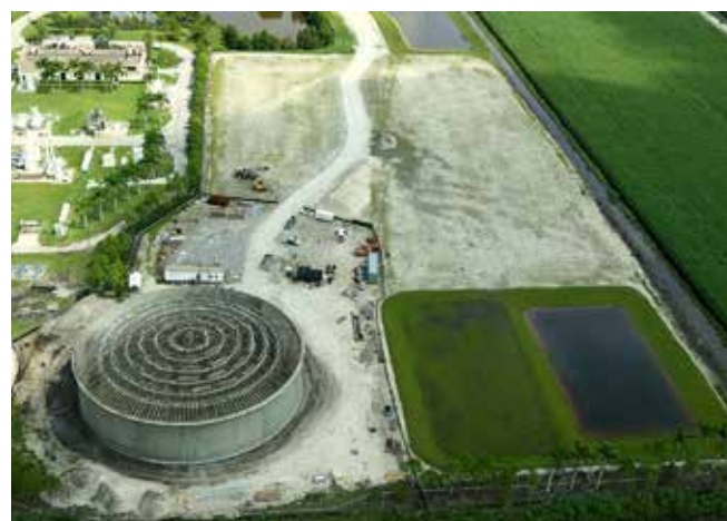
| WTP 11 New Water Storage Tank Site |
