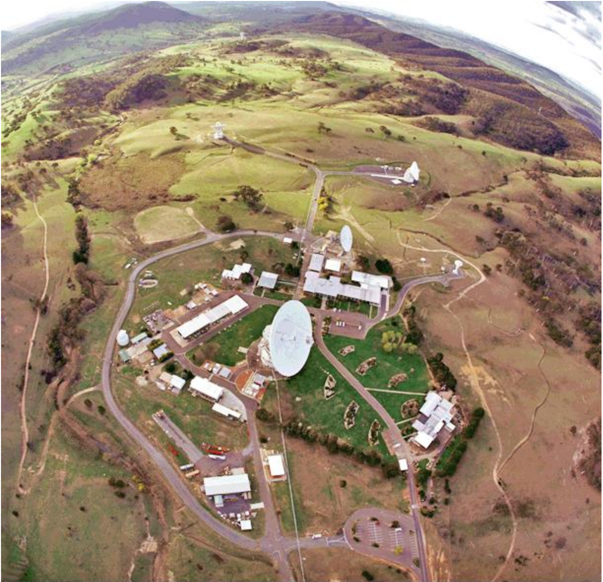
Figure 3-1. Canberra Deep Space Communications Complex (CDSCC) showing 70-m and 34-m stations.
