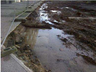
Water collecting on the exposed concrete slab of the underground car park.
