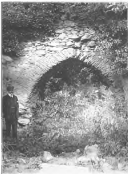
INSIDE OF OLD CHURCHTOWN CHURCH. CHANCEL.
