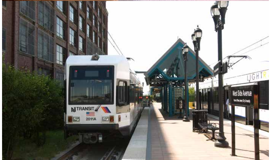
Planning to replace the outdated Portal Bridge on the Northeast Corridor (top) is underway; NJ TRANSIT is evaluating an extension of Hudson-Bergen Light Rail from this West Side Avenue Station.
