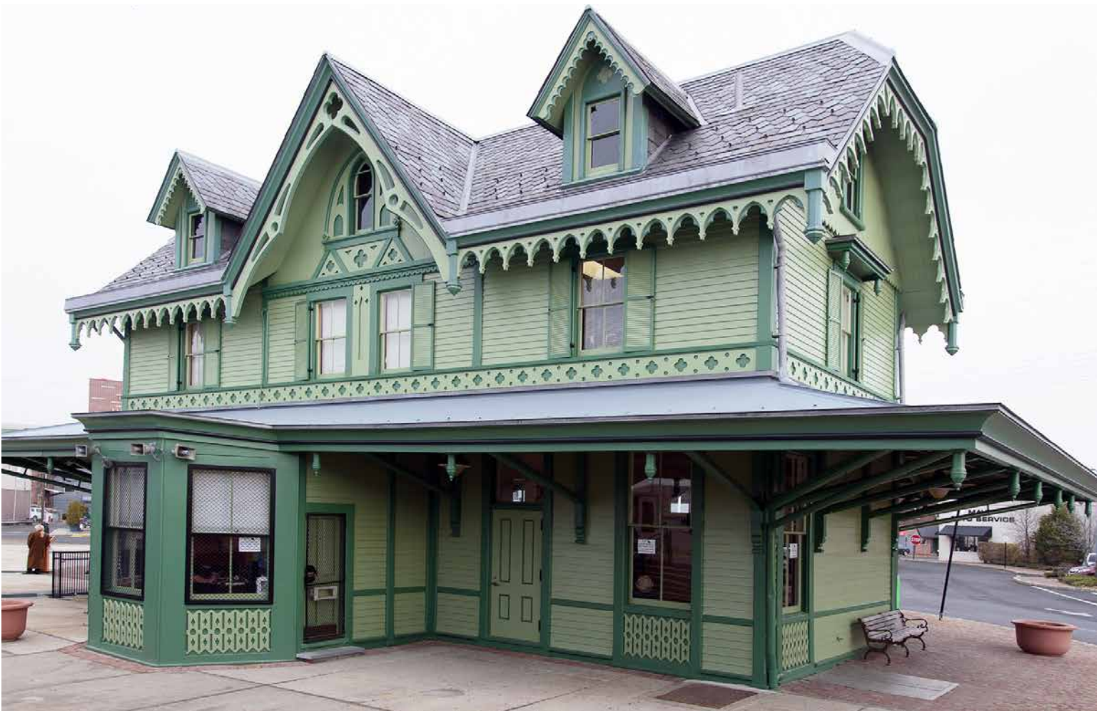
Historic Red Bank Station on the North Jersey Coast Line enjoyed a makeover in FY2015.
