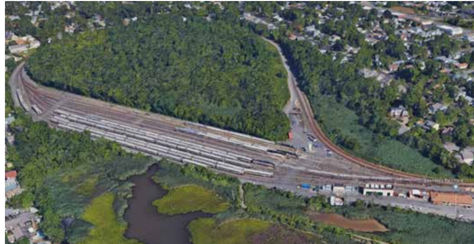
Bay Head Rail Yard
