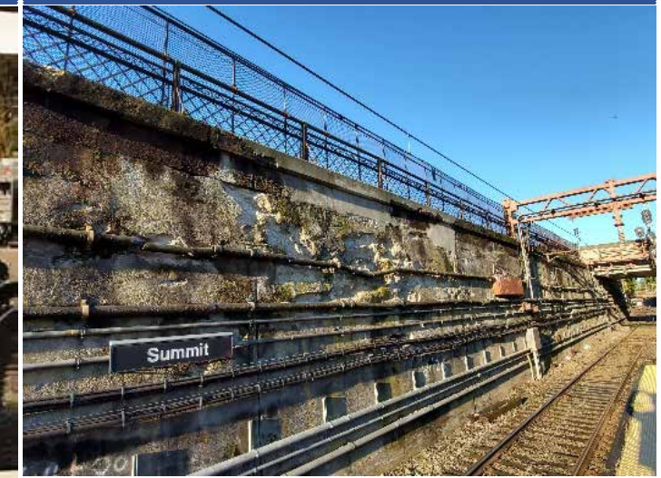
Severe Wall Deterioration
