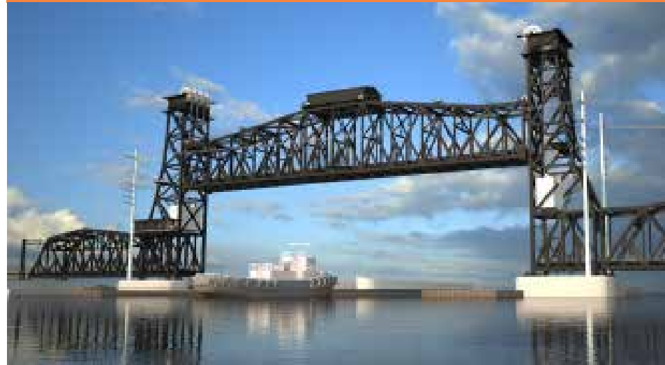
PROPOSED: New Vertical Lift Bridge
