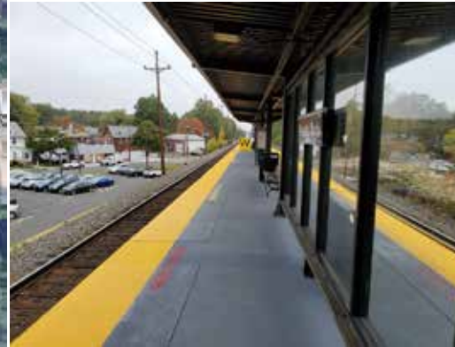
⑤ Deteriorated Platform Concrete (Typical)
