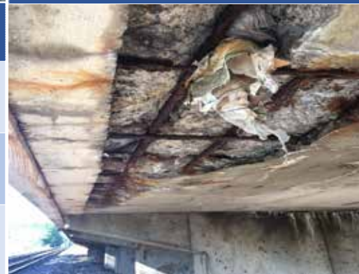
⑤ Deteriorated Platform Concrete (Typical)
