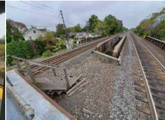
⑥ Deteriorated Platform Substructure (Typical)
