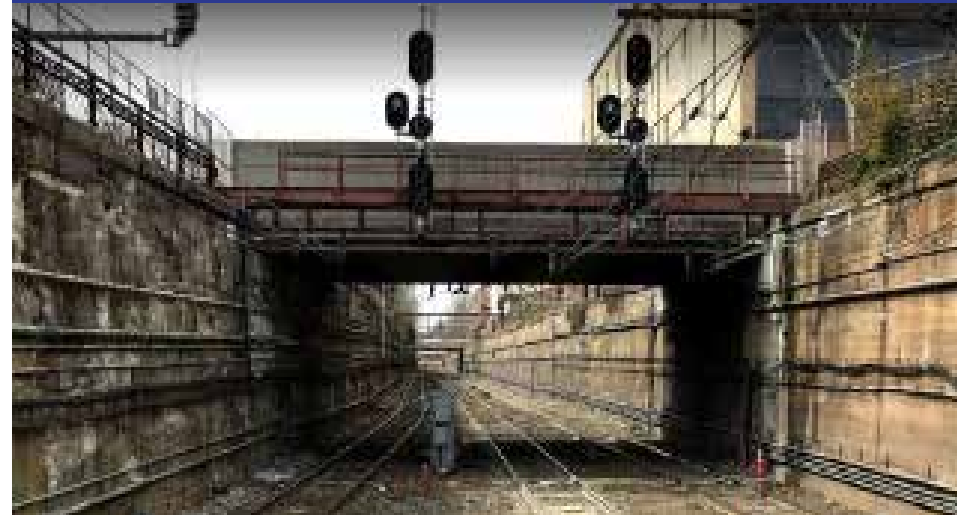
EXISTING: Overhead Bridge
