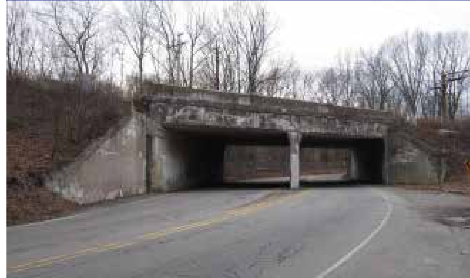
EXISTING: Undergrade Bridge
