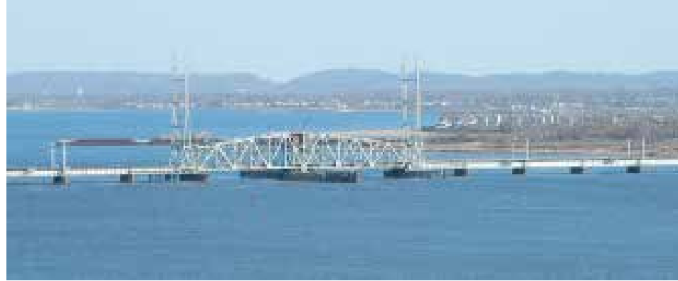
EXISTING: Swing Bridge
