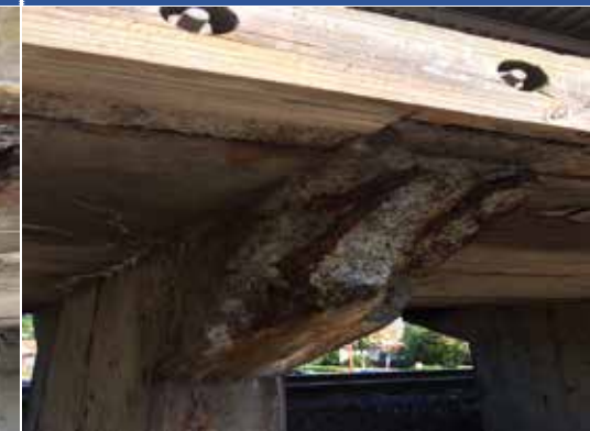
⑥ Deteriorated Platform Substructure (Typical)
