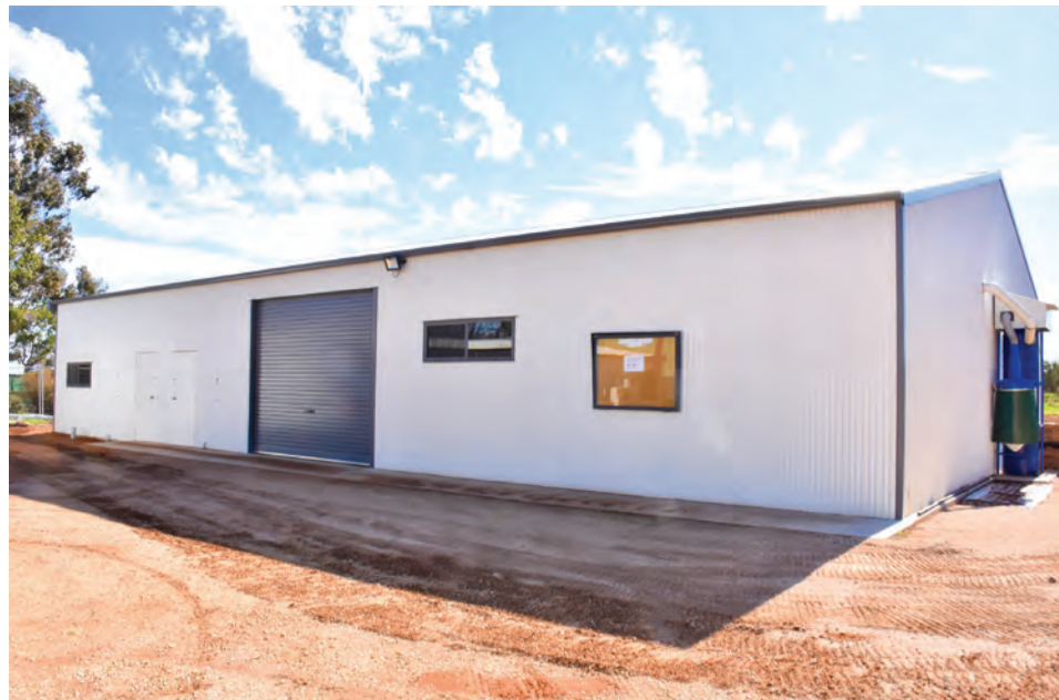
The building housing the Berri Community Men's Shed will be officially opened at a ceremony involving Berri Barmera Mayor Peter Hunt and Chaffey MP Tim Whetstone, on Sunday, November 28.
