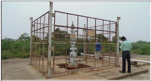
Automatic flow Oil Well near Addiyakamangalam, Thiruvapur (Location: 10°45'27.50"N 79°40'09.09"E)
