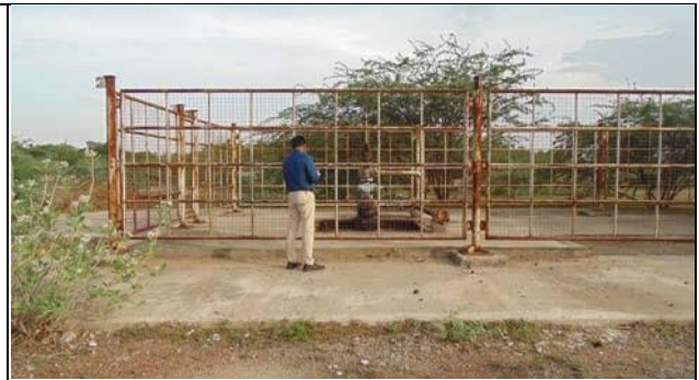
Abandoned oil well near Adhichapuram, Thiruvarur District (Location: 10°35'50.96"N 79°32'05.83"E)
