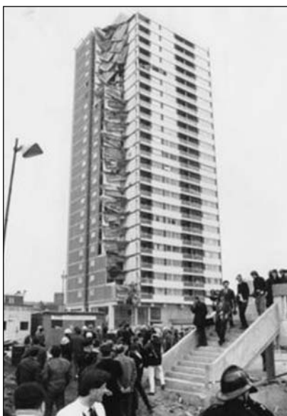
Ronan Point collapses 1968
