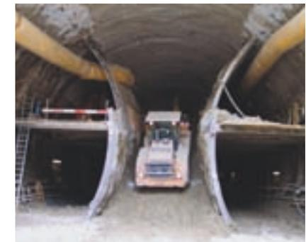
Fig. 10: core method Uettliberg
