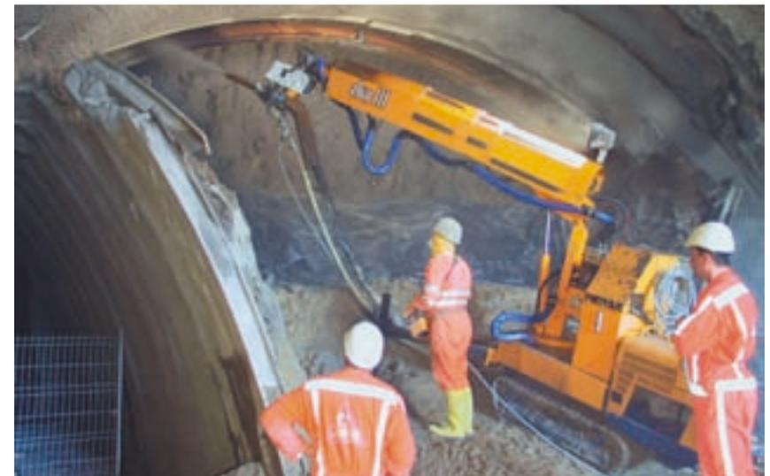
Fig. 38: sprayed concrete test for controlling rebound
