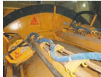
Fig. 46: Round arch spraying robot on the tunnel boring machine of the JV TAT, Gotthard base tunnel, section Bodio
