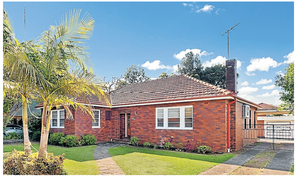
Earmarked for knock-down, this house at 22 Fernhill Avenue, Epping, was recently sold by Tracy Yap Realty for $2,116,000, $300,000 above the reserve price.
