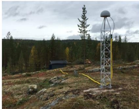
Figure 7: Typical FinnRef station ([Bhuiyan, 2022], presentation).
