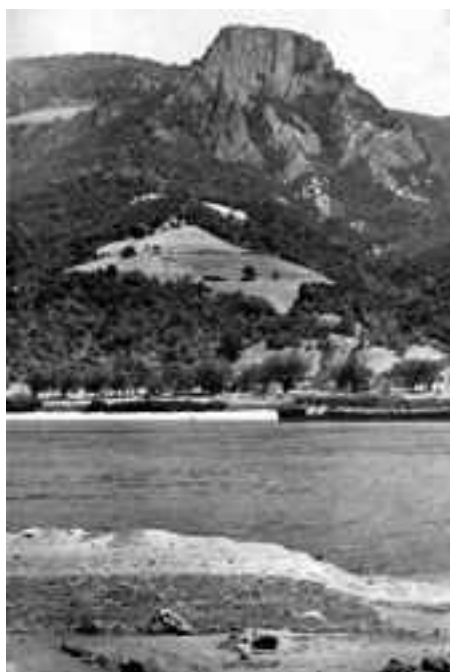
Fig. 3 Basis of the house in Lepenski Vir opposite to Treskavac – photography from [1], [2]
