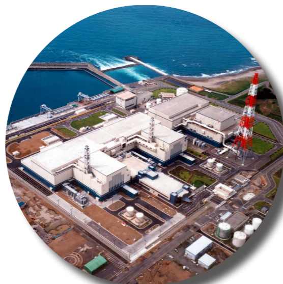
Kashiwazaki-Kariwa Nuclear Power Station, ABWR. (Kashiwazaki-Kariwa, Japan)
