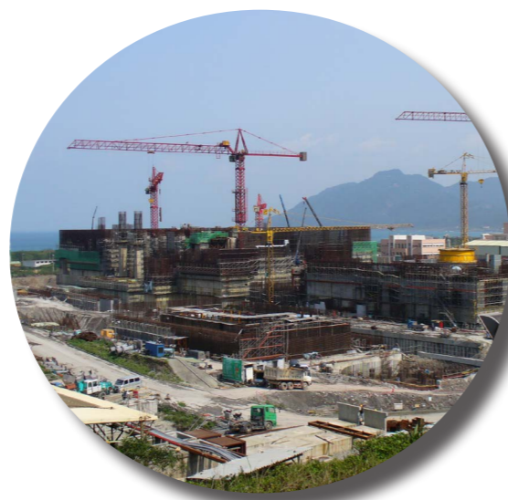
Construction of Lungmen NPP- Taiwan, China
