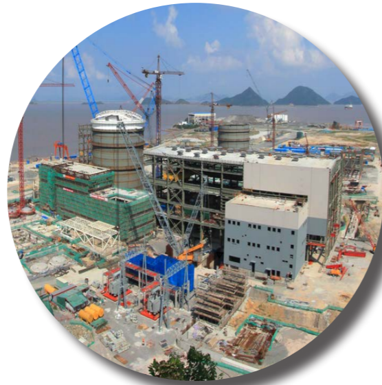
Construction Site Sanmen 1, 2 - China
