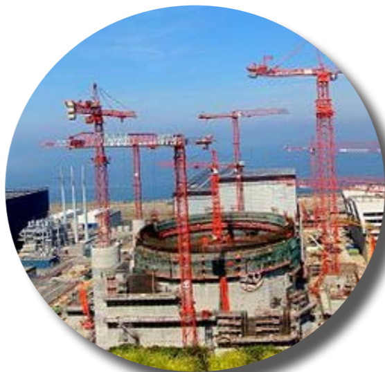
EPR Flamanville 3, France (Courtesy of AREVA)
