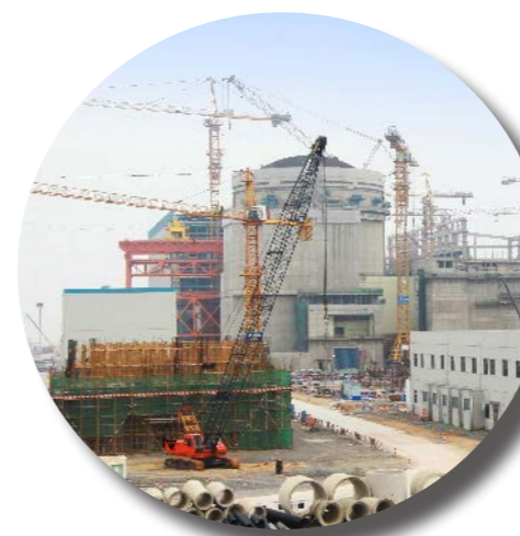
Construction of CPR-1000 at Fangchenggang, China
