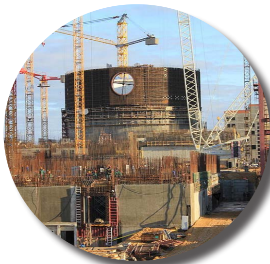
Construction of VVER1200 Novovoronezh NPP II, Russia [2]
