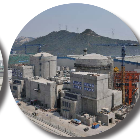
Construction of CPR-1000 and ACPR-1000 at Yangjiang, China
