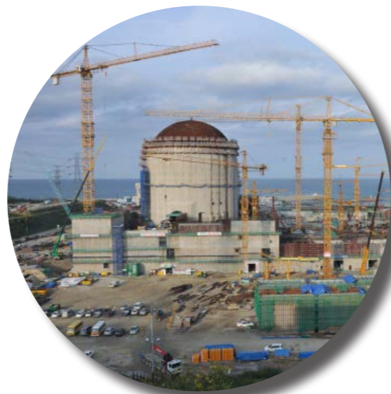
Construction of Shin-Hanul 1, Republic of Korea (Courtesy of KEPCO)
