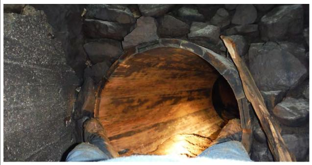
Photograph 11 Low-Level Outlet Pipe, Near Pipe Outlet
