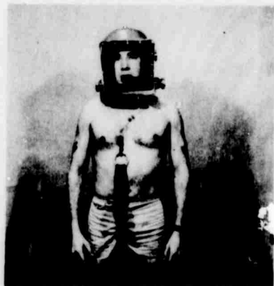
Figure 3a Front View
