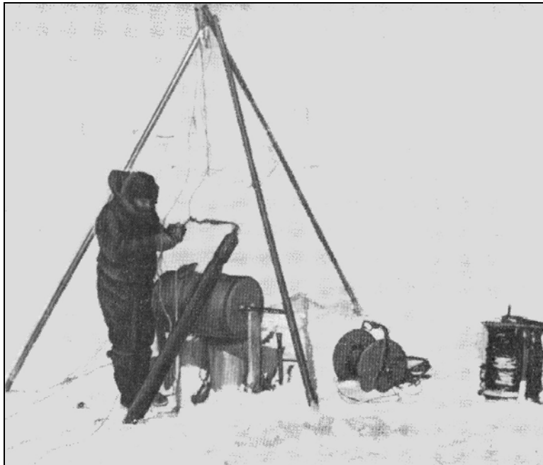
Figure 2. First experience of thermal drilling at Vostok Station during the 4 th CAE (from Ignatov 1962).
