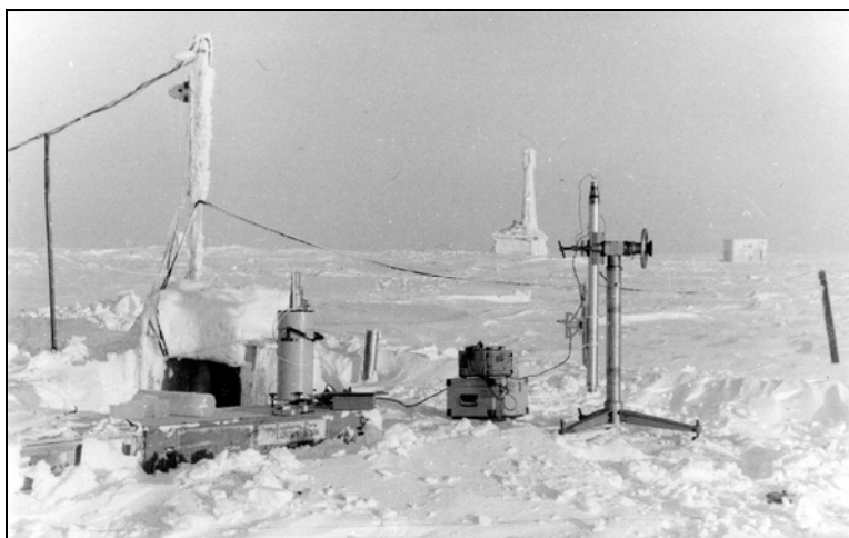
Figure 33. Calibration of directional survey tool (the drilling shelter and workshop are in the background; all living facilities were situated under the glacier surface ( Kupol Vavilova , Severnaya Zemlya, photograph by P.G. Talalay 1986)
