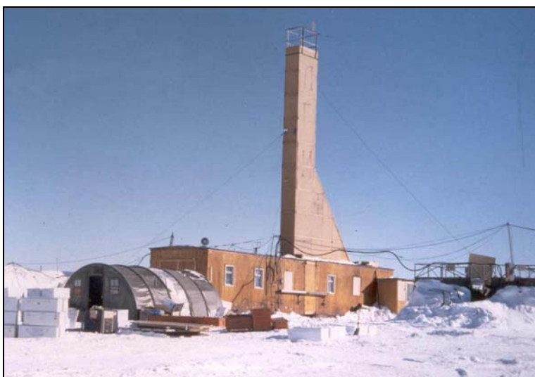
Figure 16. Drilling shelter above hole (5G) constructed during the 27th and 28th SAE (photograph by P.G.Talalay, 35 th SAE).
